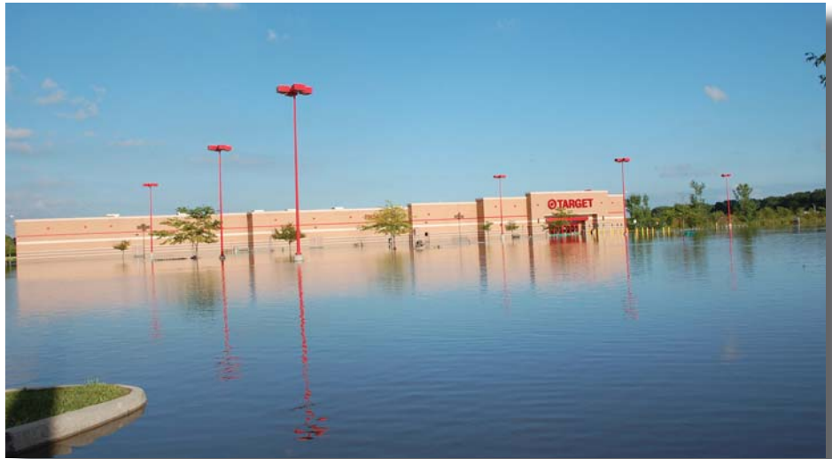
The Ames Target store was inundated by flooding of the Squaw Creek. Photo by Jace Anderson, FEMA.
