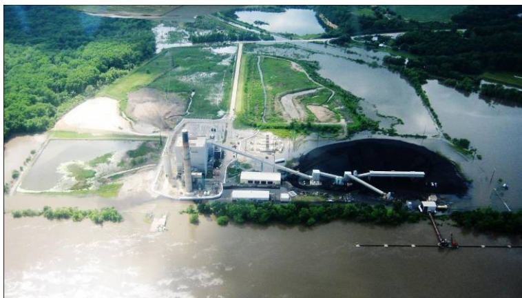
Figure 6 – Burlington's Generating Station Surrounded by Flood Waters
