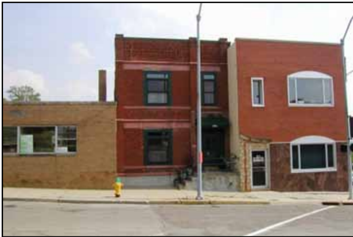
711, 709 and 707 E. Locust (left to right). 711 has already been removed. 709 and 707 will be moved or demolished so the West Capitol Terrace can be completed.
