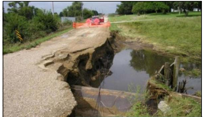
Above, a section of a gravel road in Webster County was washed out due to recent flooding. Right, the sewage lift station in Lehigh was inundated with water from the Des Moines River. Photos provided by Webster County and the Civil Air Patrol.
