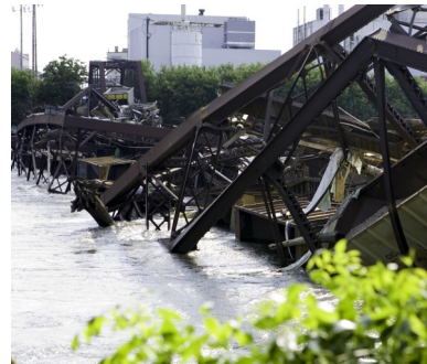
Gravel-filled railcars were not able to keep this Cedar Rapids bridge from being pulled off its pilings.
