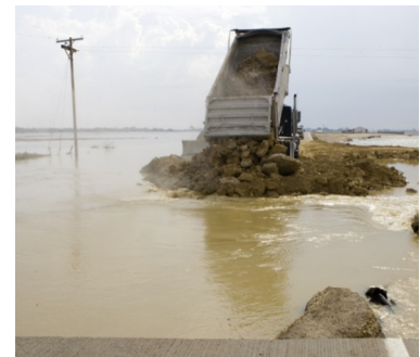
A truck dumps a load of rock into a levee breach in Oakville.
