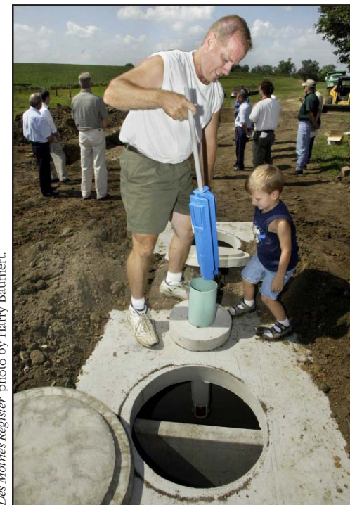
Homeowner Ken Miller, from Washington, inspects his new septic tank and effluent filter under his son's close supervision.
