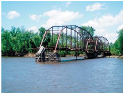
Damaged remains of the Sutliff Bridge over the Cedar River following the historic Flood of 2008.
