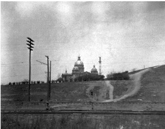
The clearing of modest structures and enhancement of the south axis greatly improved views from the trunk line trains.
