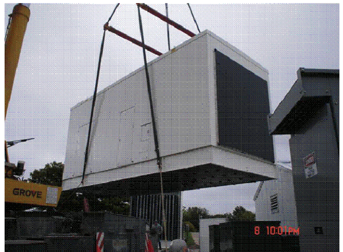
Contractors lifting new generator in place. This unit weighed in at 66,000 pounds!
