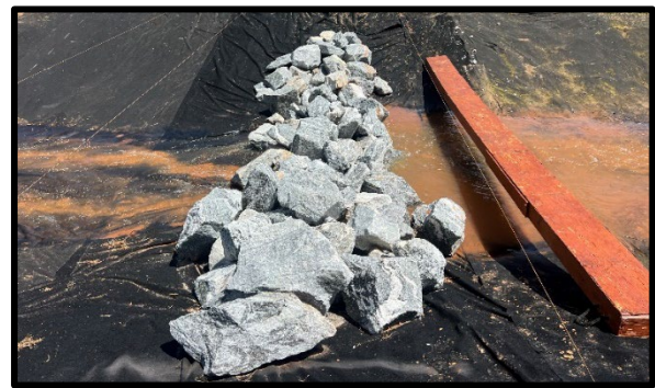
Performance of Installation On Grade
