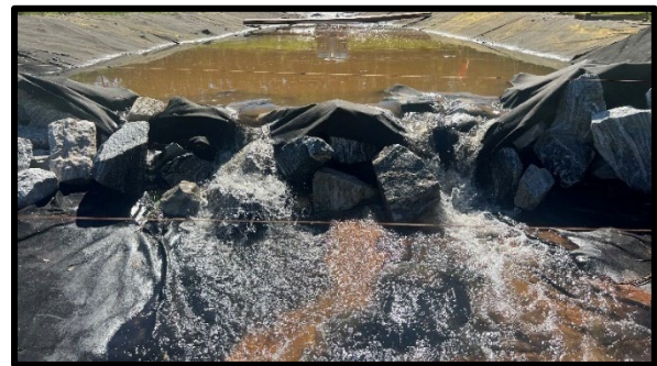
Large Rock Overtopping at Low Points
