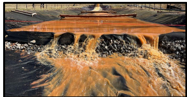
Most Feasible and Effective Installation (MFE-I) overtopping
