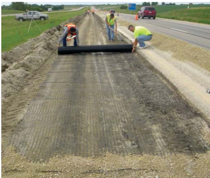
Rolling the geogrid over the soft subgrade layer near Nashua, Iowa
