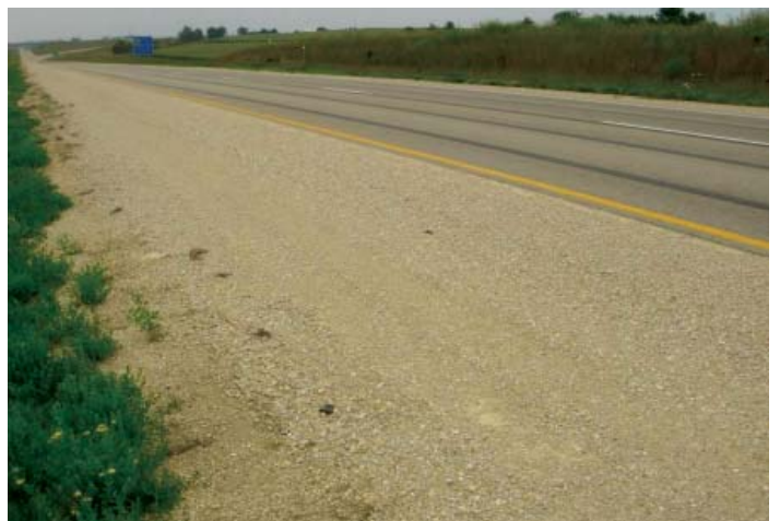
Inside shoulder near Nashua, Iowa: before stabilization (top) and two months after stabilization (bottom)
