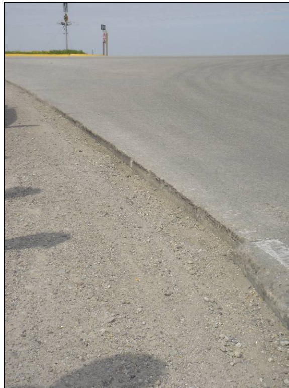
Figure 37. Granular shoulder section at exit ramp of Hwy 65 onto Hwy 27, May 10, 2006
