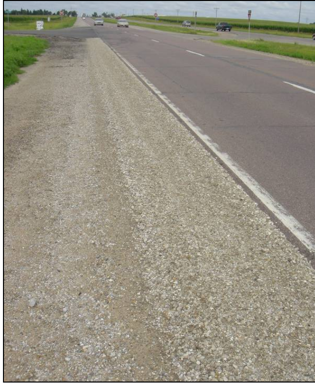
Figure 43. Granular shoulder section on Hwy 122, July 26, 2005
