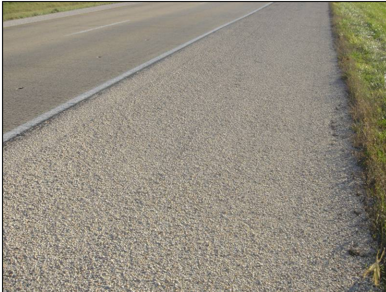
Figure 97. FA surface sealed using chip seal on I-35 milepost 150 northbound, September 1, 2005
