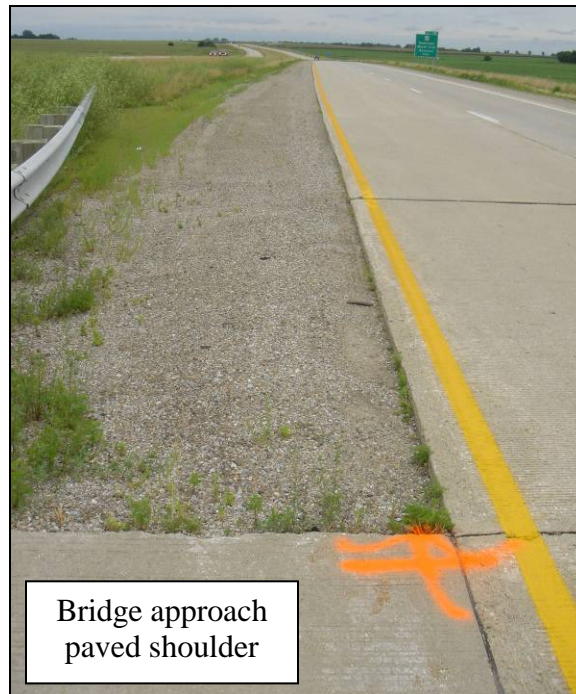
Figure 17. Granular shoulder section following a paved bridge approach shoulder, Hwy 18 milepost 184.55 E.B., July 26, 2005
