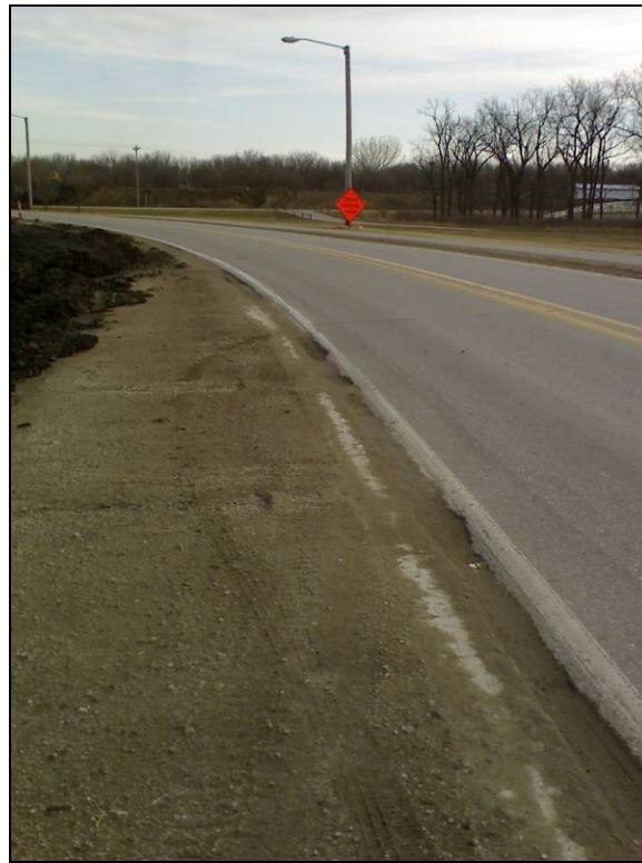
Figure 130. Significant edge drop-off observed after four months on 16th St. Ames, IA, December, 2007
