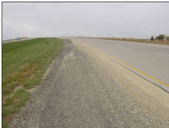
Figure 117. Asphalt millings placed at the shoulder test section and a 2 in. edge drop-off developed after two months, October 10, 2006
