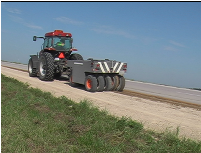
Figure 113. Compacting the stabilized section using a pneumatic roller on Hwy 18 milepost 202.50 Rudd, IA, on August 22, 2006
