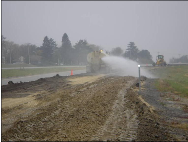
Figure 150. Water truck used to increase moisture content of clay-fly ash mixture, October 31, 2005
