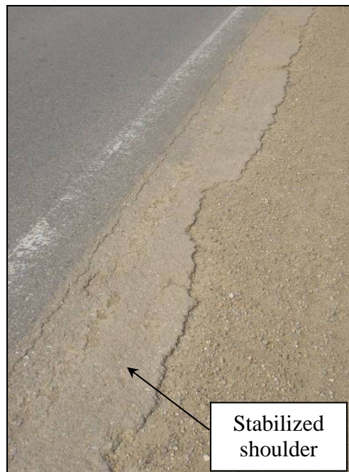
Figure 25. Granular shoulder section stabilized with soybean oil, May 10, 2006
