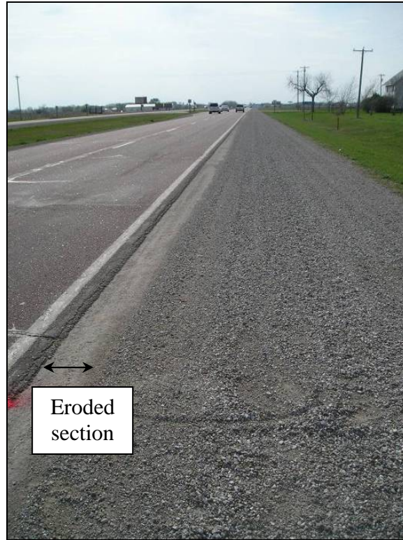
Figure 82. Erosion of the granular shoulder adjacent to the pavement edge on Hwy 122, April 18, 2005
