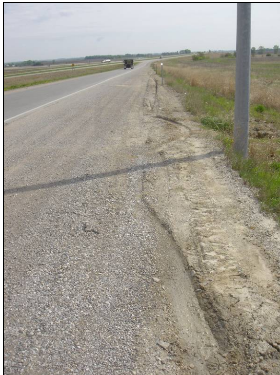
Figure 39. Shoulder rutting caused by soft subgrade and absence of granular layer on Hwy 65 exit ramp to Hwy 27, May 10, 2006
