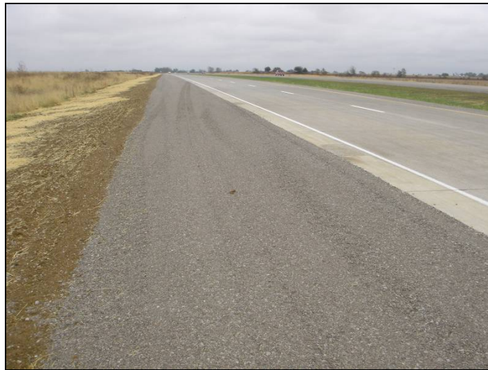
Figure 162. Newly constructed granular shoulder section, October 17, 2006
