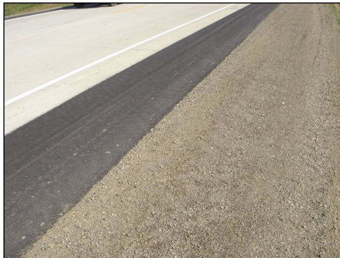
Figure 71. Shoulder section with 4 ft. of HMA and 4 ft. of blended limestone and crushed concrete on Hwy 60 St. 149+00', October 14, 2005
