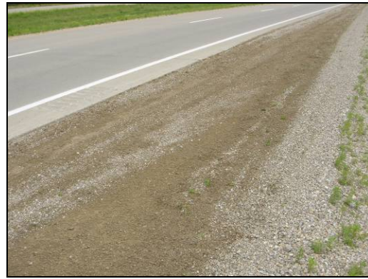
(b) Shoulder surface after blading
