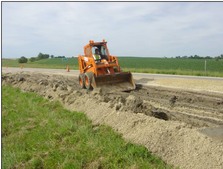
Figure 173. Skid loader leveling the subgrade, June 23, 2006
