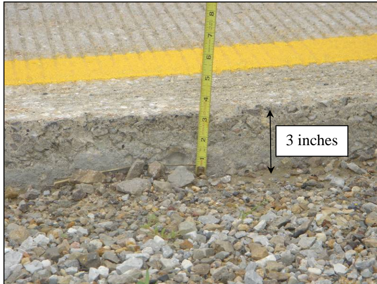
Figure 18. Three-inch shoulder drop-off, Hwy 18 milepost 184.55 E.B., July 26 2005
