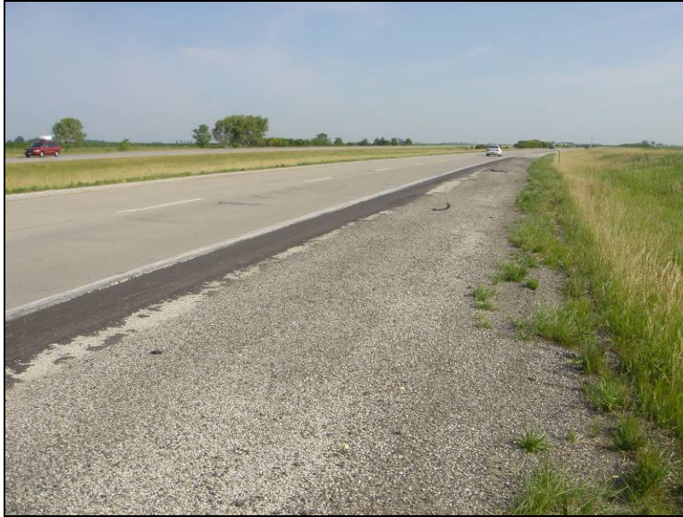
Figure 103. Asphalt patch placed on the deteriorated shoulder adjacent to a horizontal curve, I-35 milepost 150 northbound, July 7, 2006
