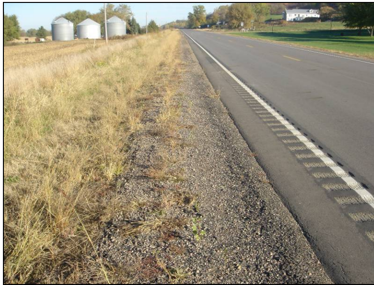
Figure 52. Granular shoulder section (southbound shoulder looking north) on Hwy IA 12 Station 1080+00', October 14, 2005
