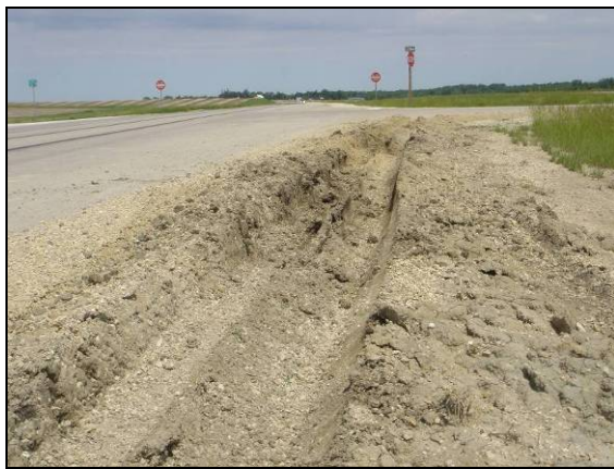
(a) Rutting extending to the underlying clay layer
