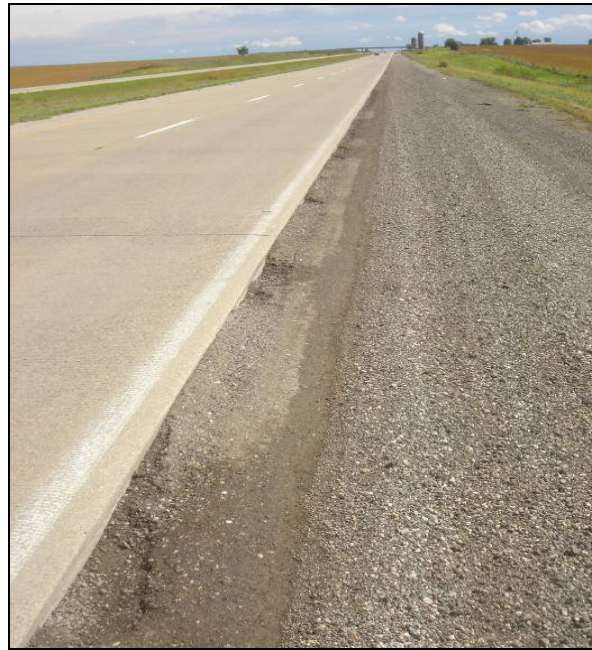
Figure 47. Granular shoulder section maintained with asphalt millings on Hwy 20 milepost 242 E.B., September 23, 2006
