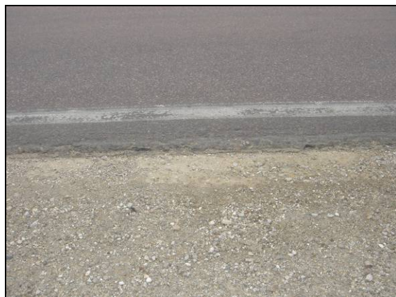
(a) Delaminated strip near pavement edge
