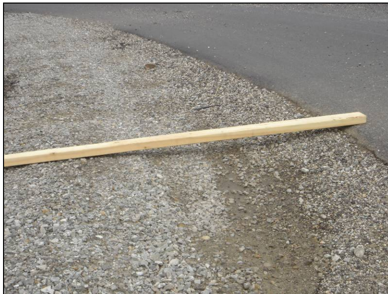
Figure 44. Cross slope damage at the intersection with Larke Ave. on Hwy 122, July 26, 2005
