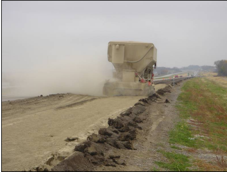
Figure 148. Semi trailer bottom dump truck spreading fly ash on top of subgrade layer, October 31, 2005
