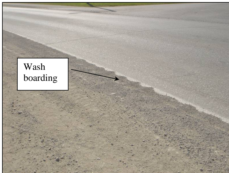
Figure 128. Development of wash boarding towards the end of the section (seven days after construction), October 3, 2006
