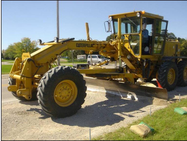
Figure 122. Blading of the shoulder section on 16th St. in Ames, IA, September 26, 2006
