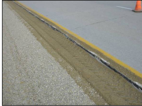
(b) Tilled granular layer to a depth of 6 in.
