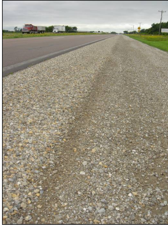
Figure 90. Crushed limestone added to areas with high edge drop-off on Hwy 122, July 26, 2005
