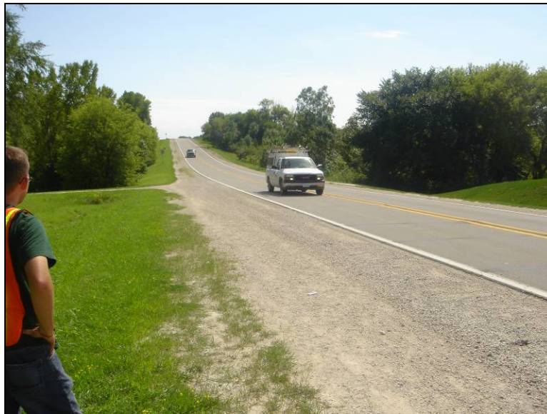
Figure 76. Aggregate shoulder section on State Ave., August 19, 2005
