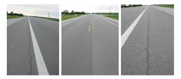
Figure 9-5. Longitudinal cracks created along the shoulder of both lanes
