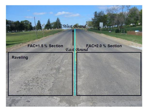
Figure 10-16. Comparison of CIR-foam pavement raveling at two different FAC
