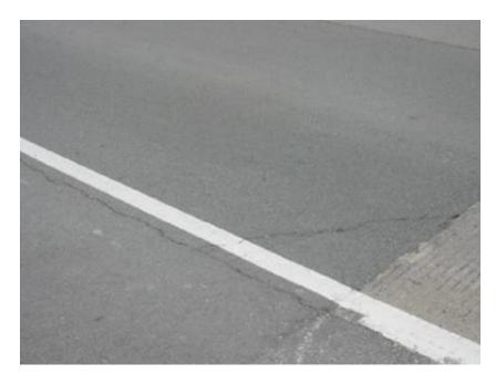
Figure 9-4. Longitudinal and transverse cracks at the interface between rehabilitated pavement and un-rehabilitated pavement
