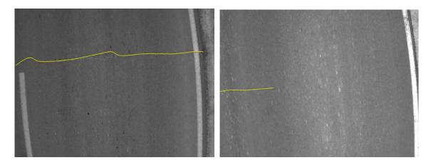
Figure 9-6 Transverse crack patterns measured from Webster County
