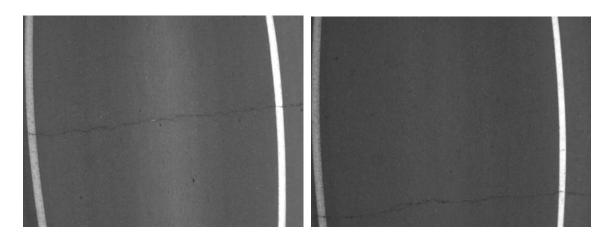
Figure 9-8. Transverse crack patterns measured from Hardin Countyd
