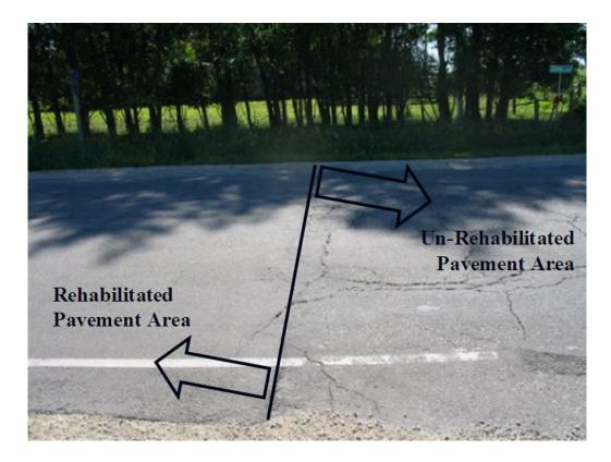
Figure 9-12. Cracks created at the interface between rehabilitated pavement and unrehabilitated pavement
