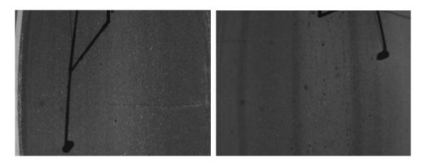
Figure 9-10. Longitudinal and transverse cracks measured from Montgomery County
