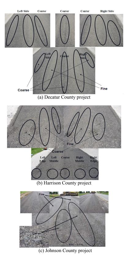
Figure 10-13. Pictures of paved foamed asphalt mixtures observed from CIR-foam field projects
