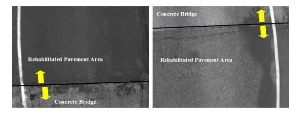
Figure 9-9. Alligator cracks at the interface between rehabilitated pavement and existing concrete bridge.
