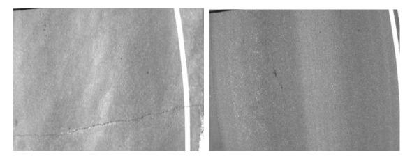
Figure 9-11. Longitudinal and transverse cracks measured from Bremer County
