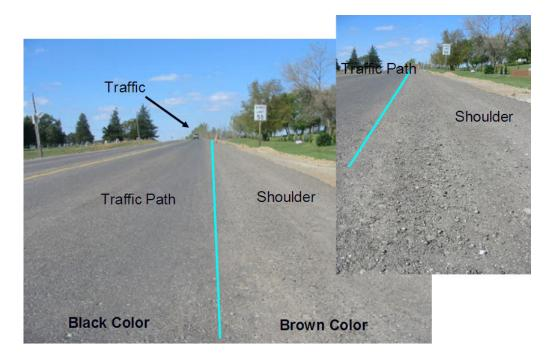
Figure 10-17. Comparison of CIR-foam pavement between traffic path and shoulder
