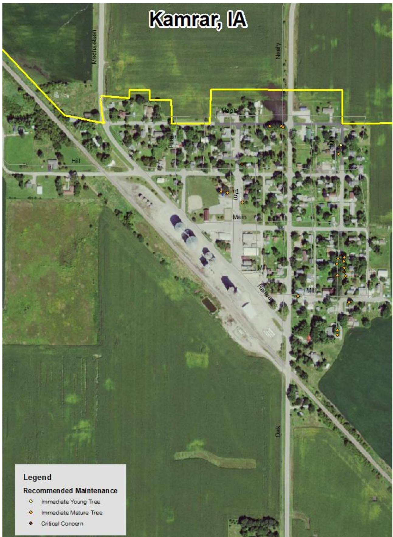
Figure 4: Location of Trees with Recommended Maintenance
