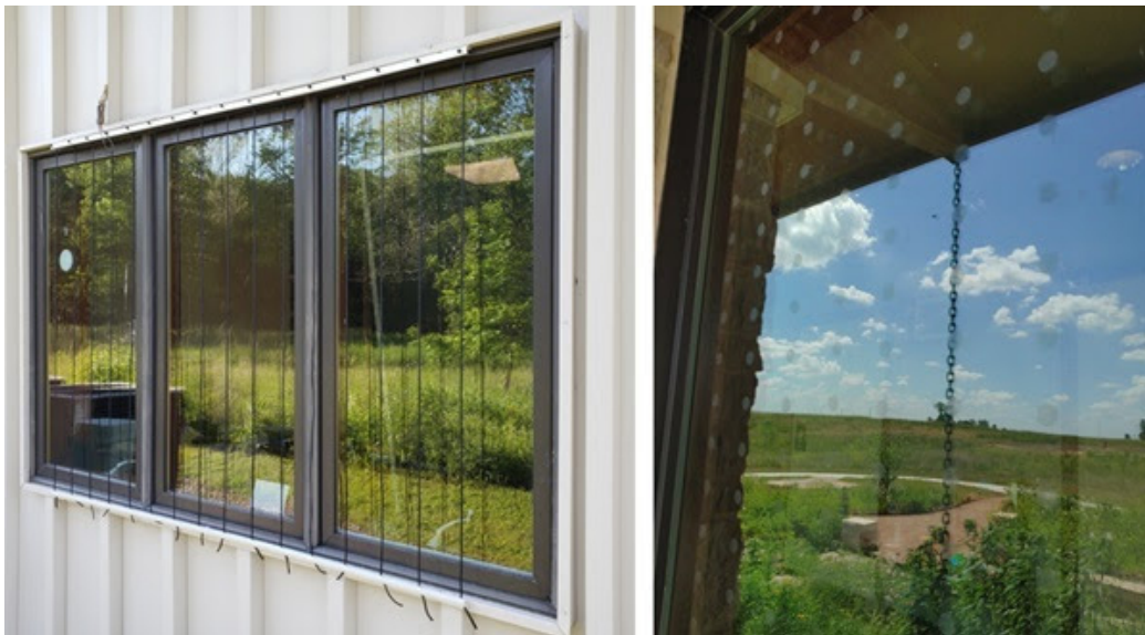
Windows with parachute cord blinds (left) or ultraviolet tape (right) can help prevent bird window collisions.
