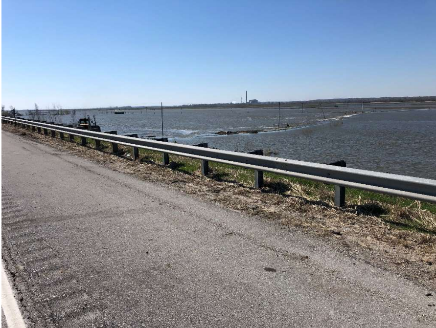
Figure 3. Photograph of SENSr System Deployed on I-29 Bridge
