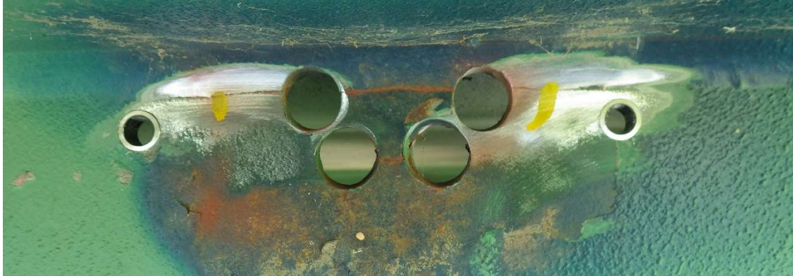
Figure 4 – installation on bridge 6724.7S141
