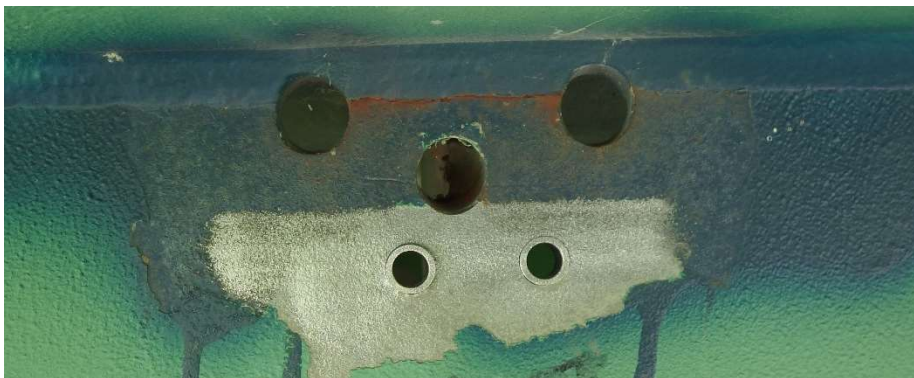
Figure 5 – second installation on bridge 6724.7S141
