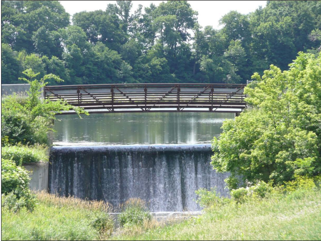
Figure 2-5. Ogee spillway at northwest corner of Briggs Woods Lake.
