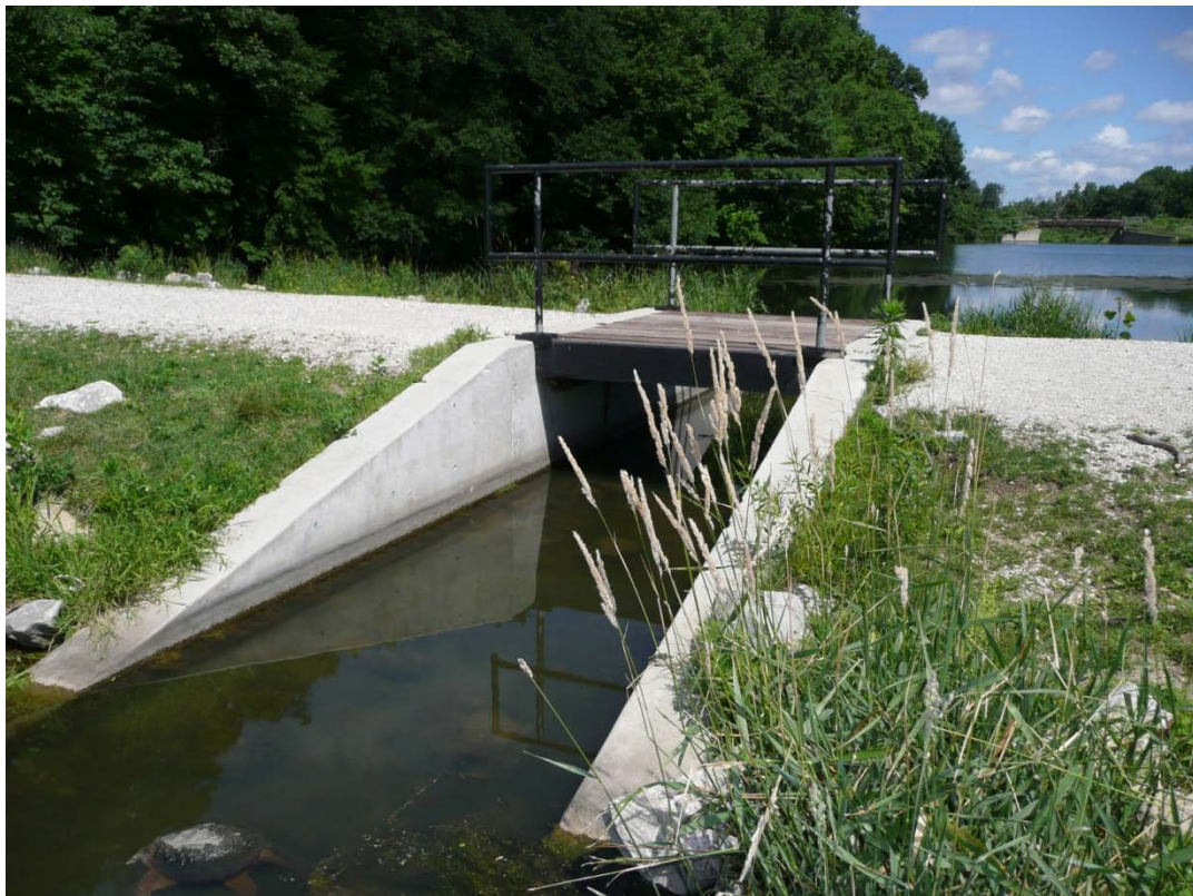
Figure 2-6. Culvert/weir passing low flow through diversion berm.
