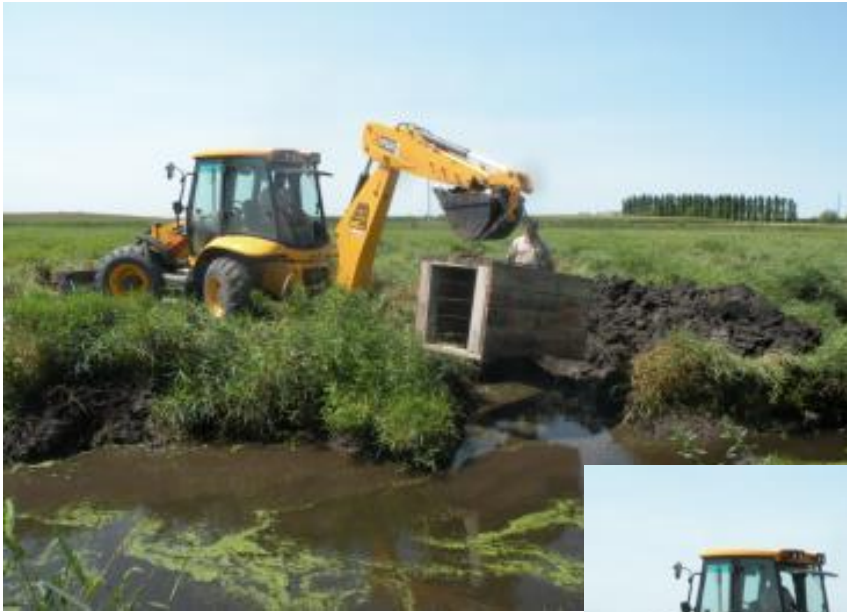
Figure 11- 18. Turtle Hibernaculum. In the winter reptiles must hibernate underground or underwater to prevent their bodies from freezing. This wooden structure provides a secure wintering area for turtles.
