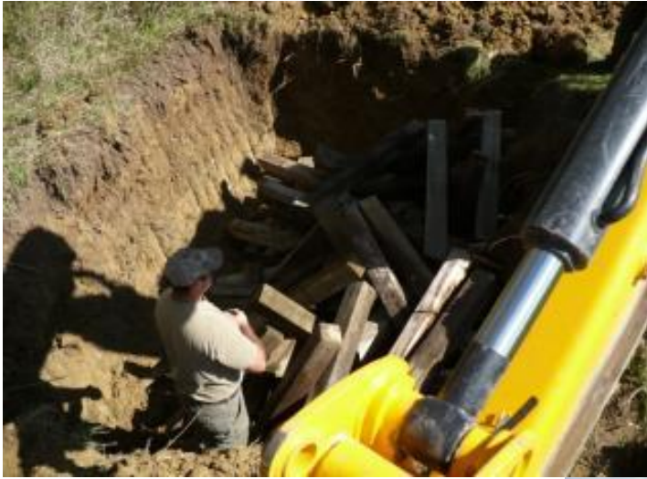
Figure 11- 16. Hole dug at McCoy WMA that was filled with logs to provide a hibernaculum for snakes (above). The hole was filled and the south side was covered with rock to provide an entrance (below).
