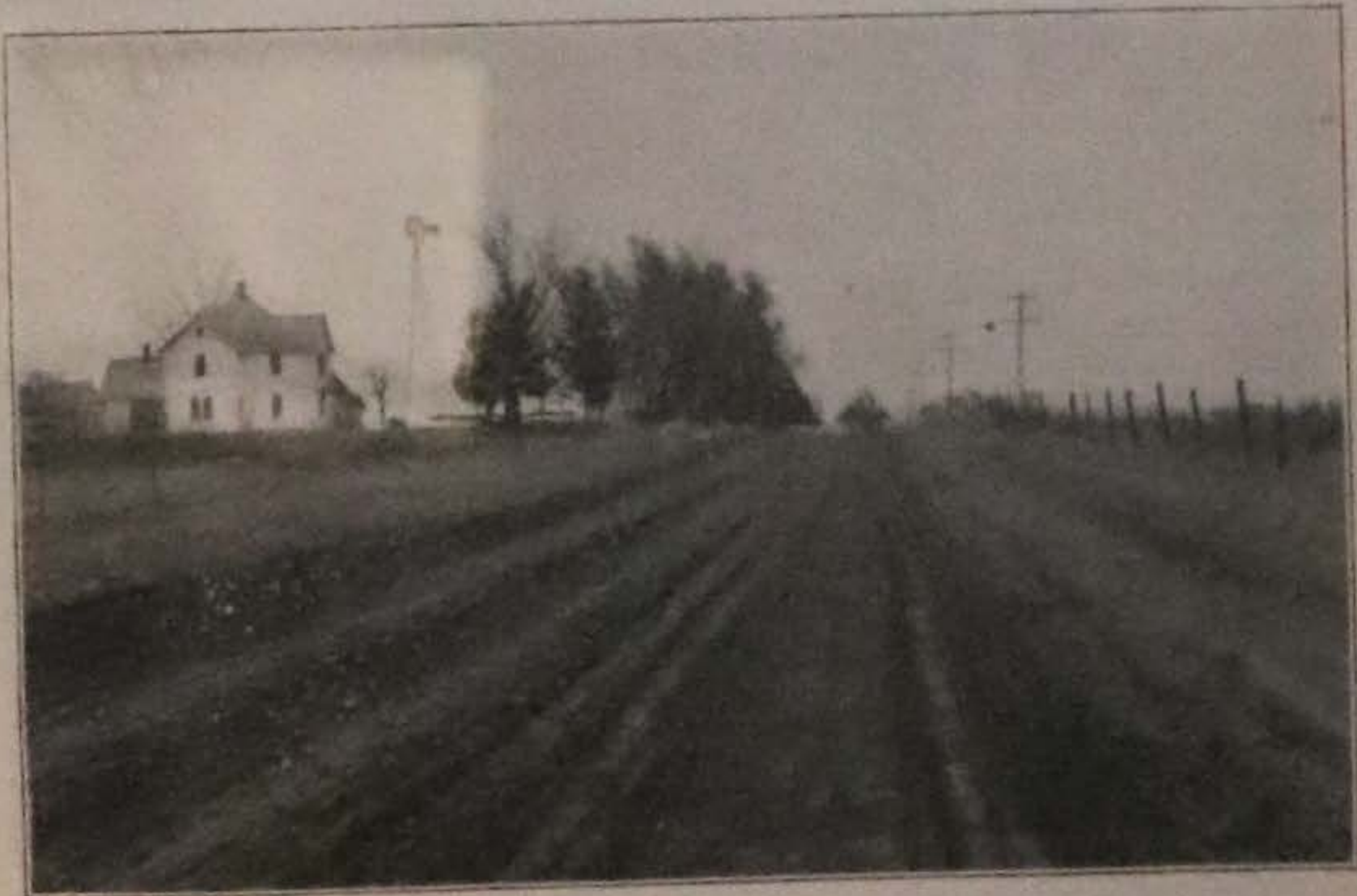
Figure 21. April 7, 1900. This view was taken the same date as Figures 22 and 23, which are nearby roads. The value of dragging is clearly apparent. This is a portion of road shown in Figure 23.
