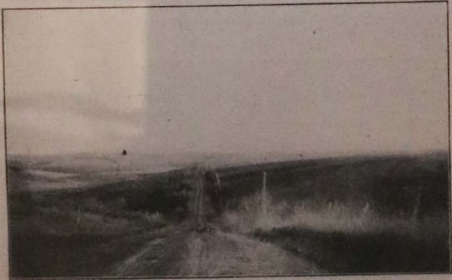
Fig. 7—SECTION LINE LOCATION This road parallels a valley which is proper location for the road.
