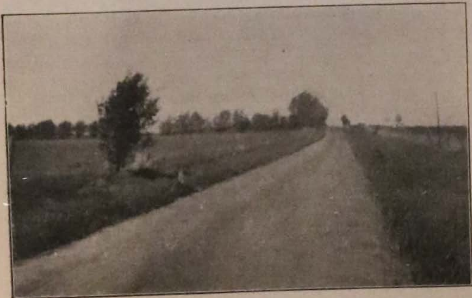
Figure 30. Gravel Road in Carrol County. This road has been maintained by the drag method.
