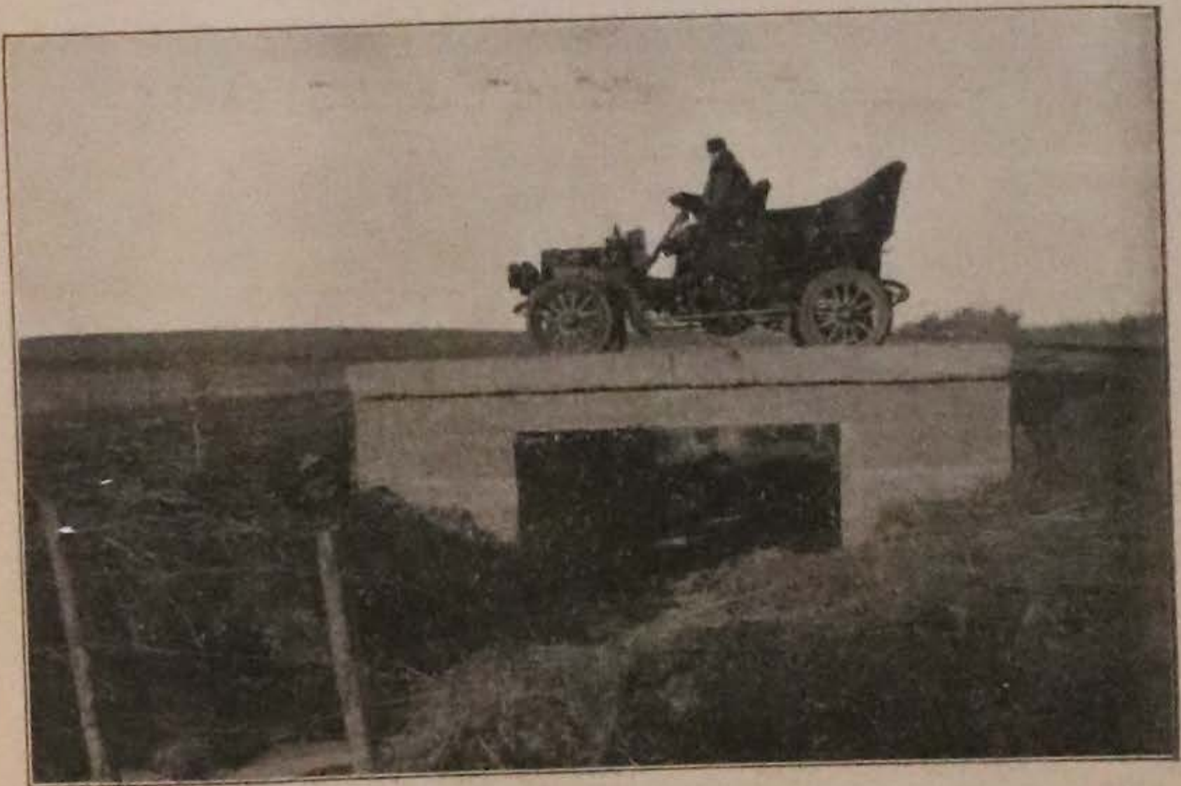
Fig. 34—Flat Top Culvert near Jefferson, Iowa.
