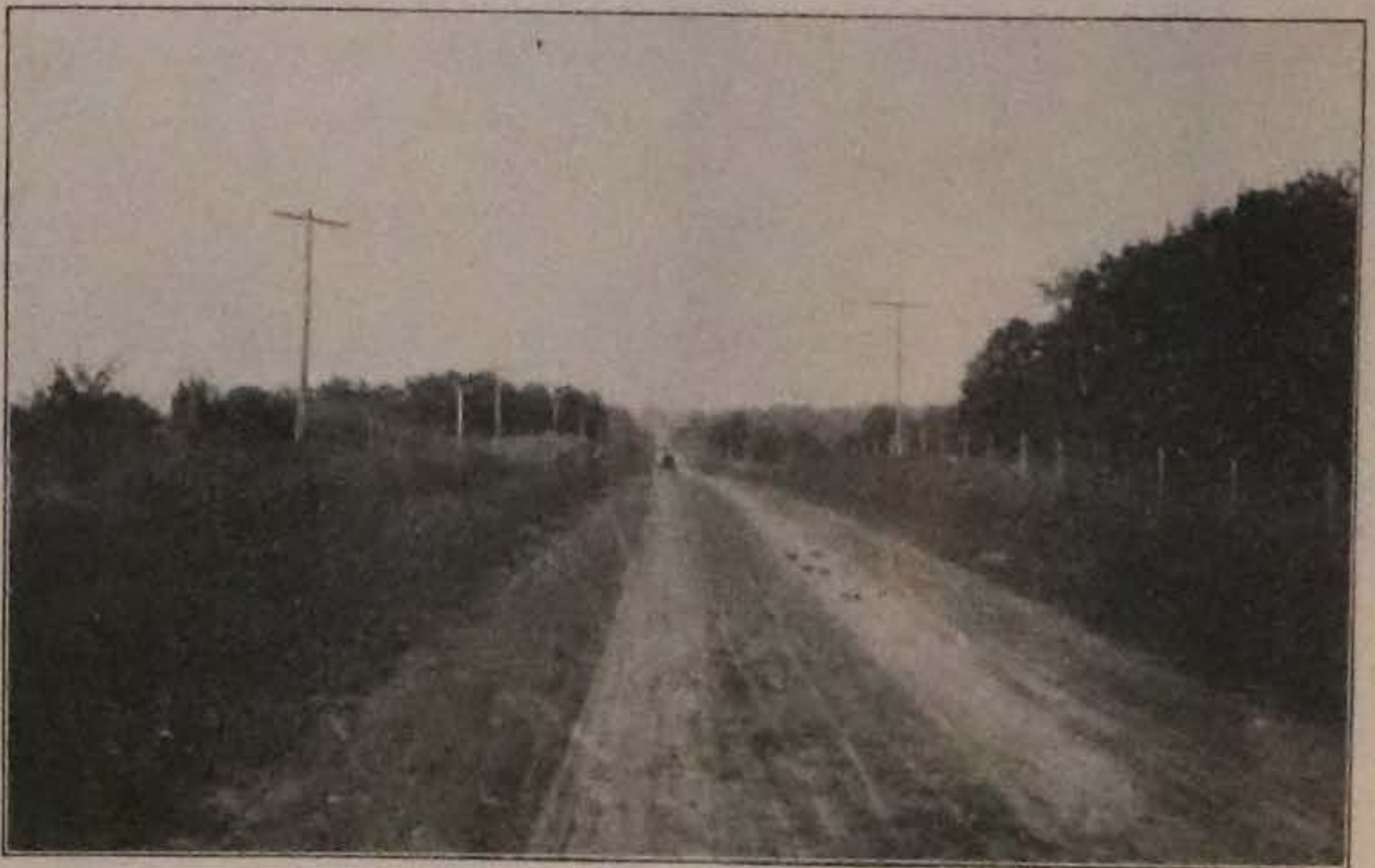
Fig. 14—A Well Built Gravel Road in Greene County
