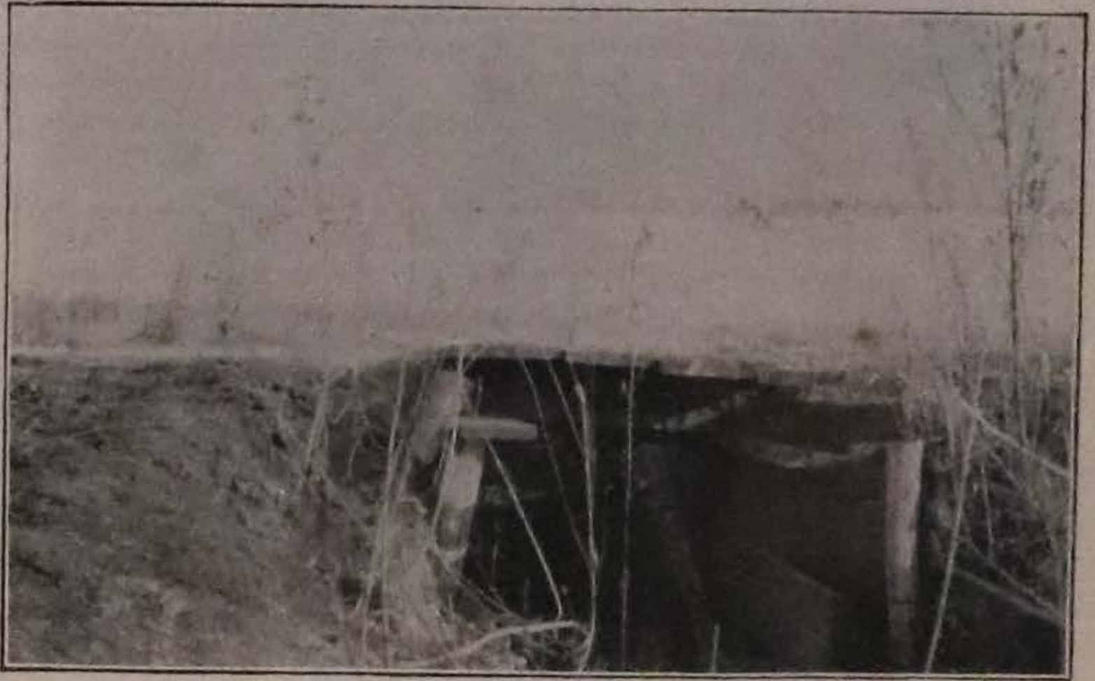
Fig. 37—A Typical Timber Culvert in Typical Condition
