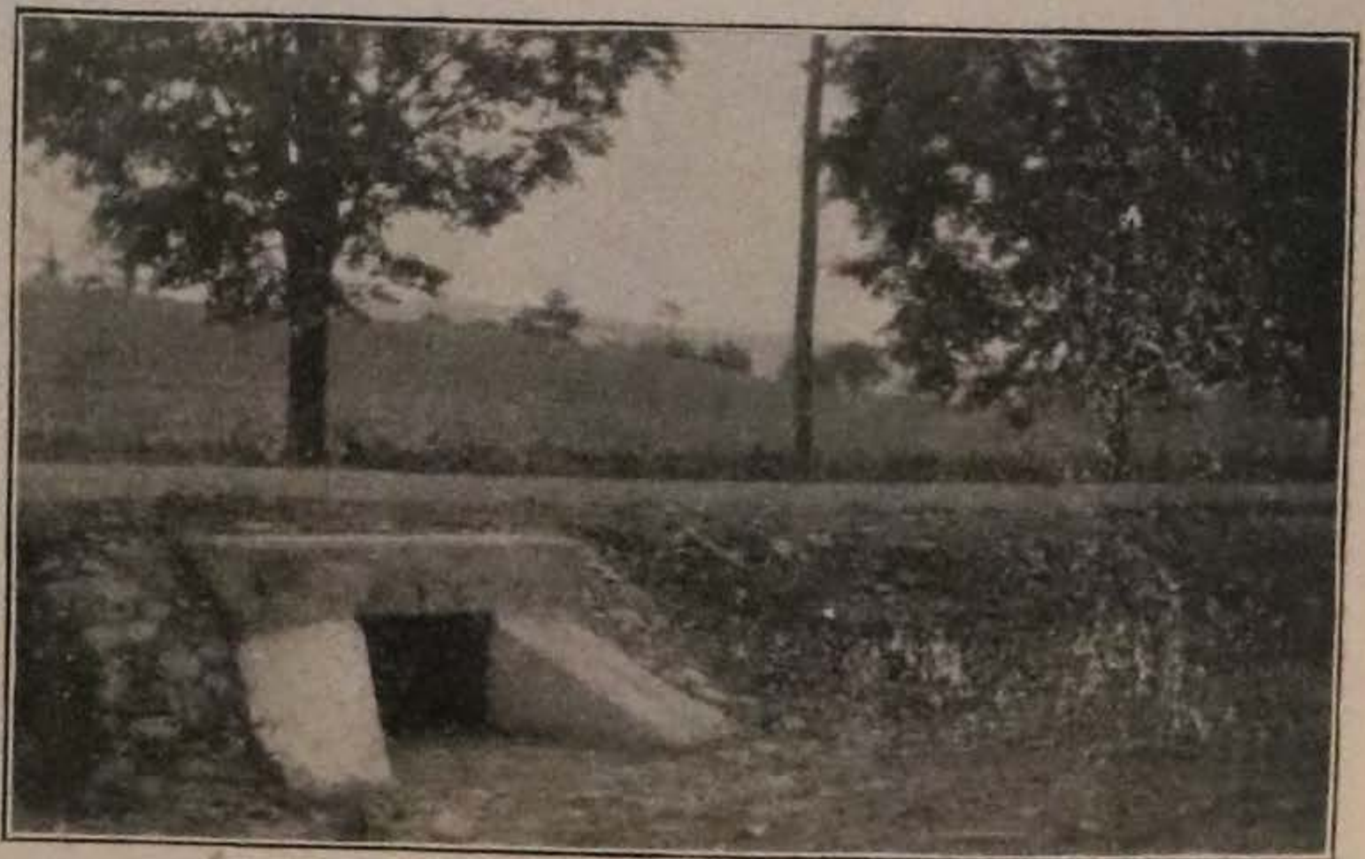
Fig. 38—A Reinforced Concrete Culvert now in common use in the Eastern States
