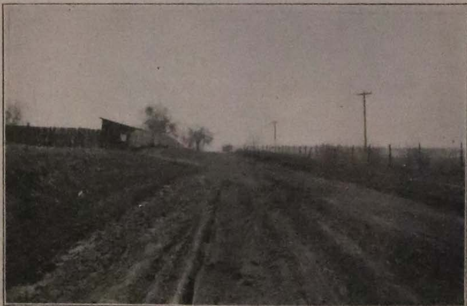
Figure 24. April 27, 1906. "On the upper Iowa City road from Tipton near the Fair grounds. The road is dry, rutty and rough. In the foreground the travel is close to the fence on the north side of the road, but soon crosses to the south side going on the bank close to the sheds."
