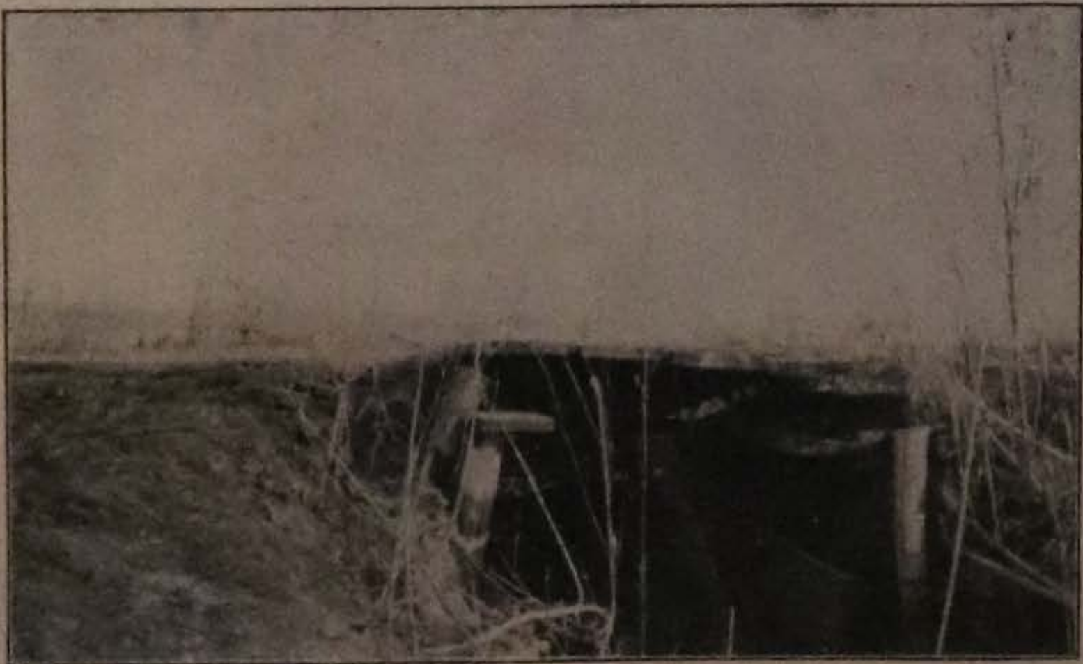
Fig. 22—A TIMBER CULVERT IN TYPICAL CONDITIONS
