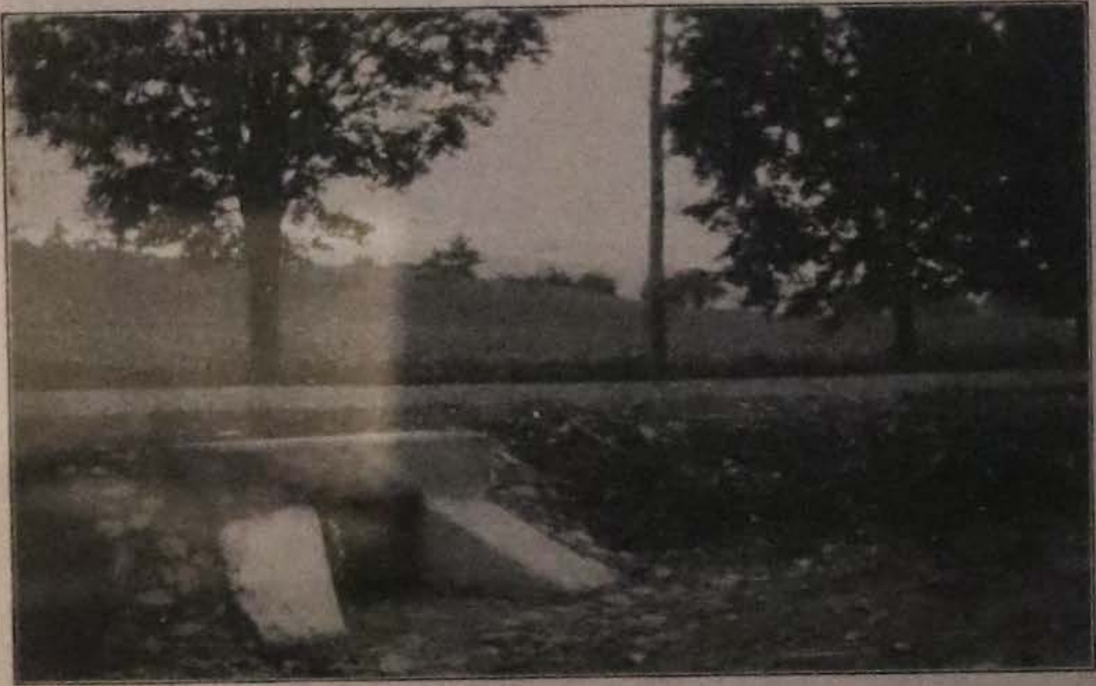
Fig. 24—A CONCRETE CULVERT IN PLACE This is practically indestructible.
