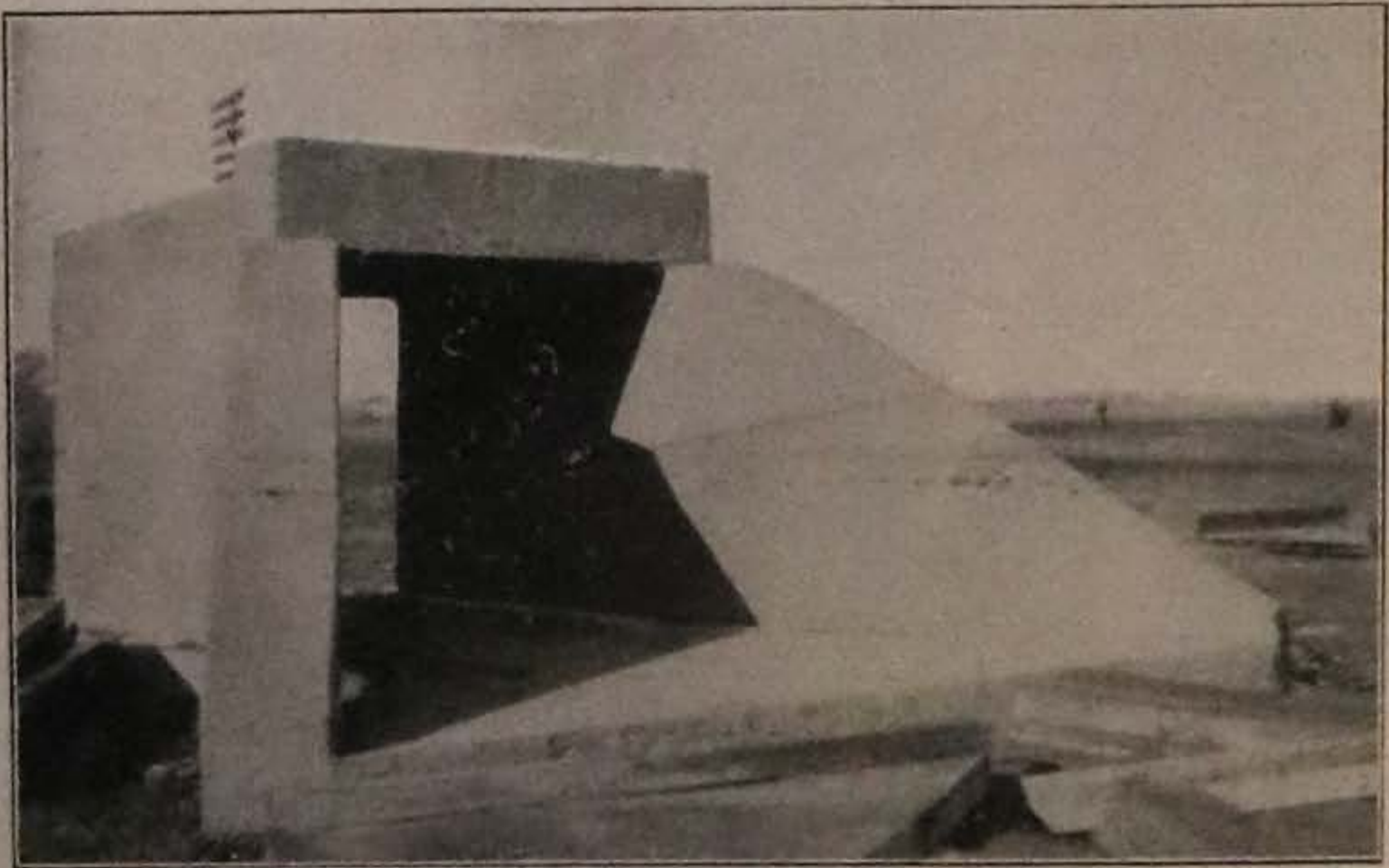
Fig. 23—TEST CULVERT OF IOWA HIGHWAY COMMISSION, AMES, IOWA
