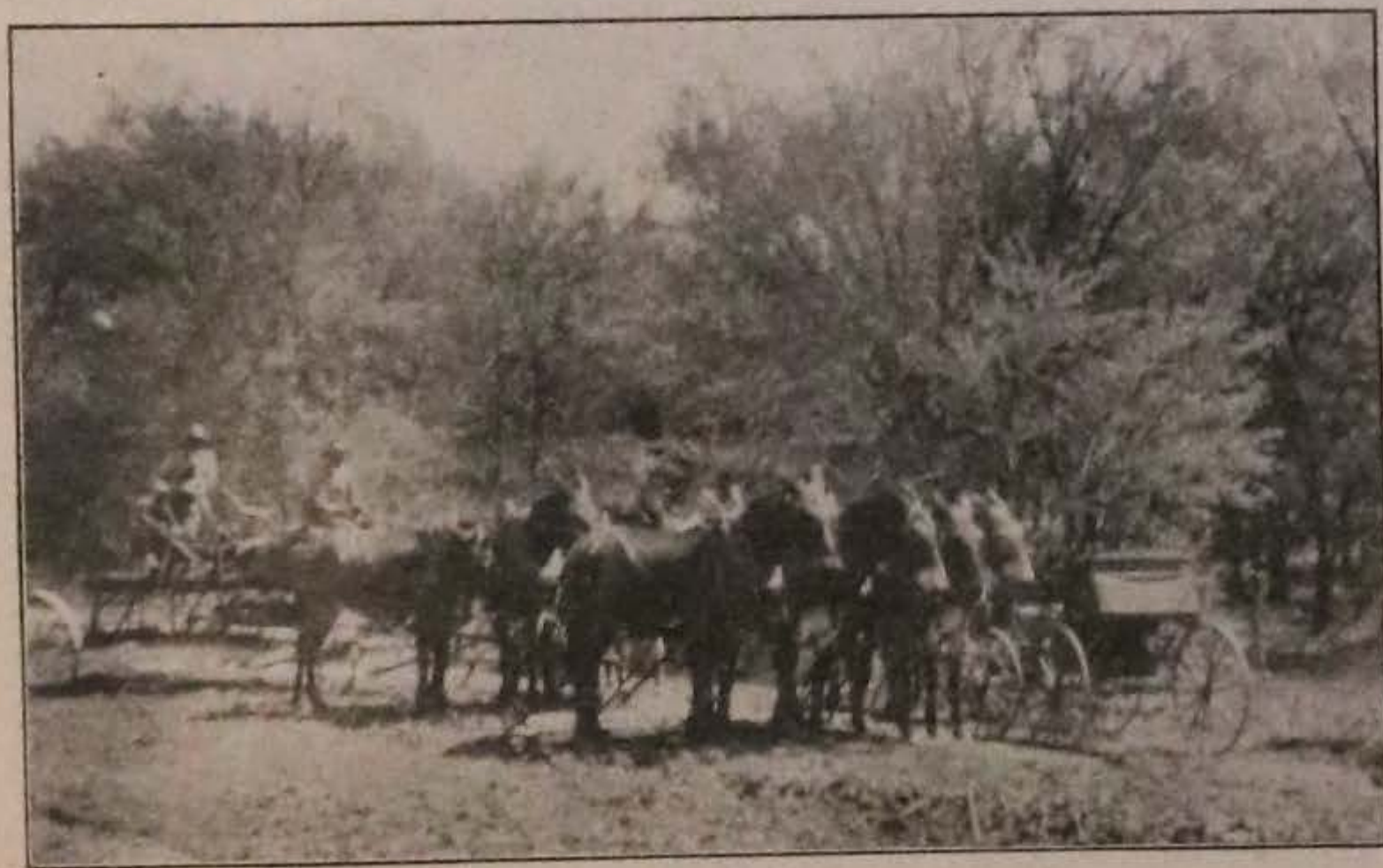
Fig. 11—AN EFFICIENT WELL TRAINED TEAM FOR ROAD BUILDING
