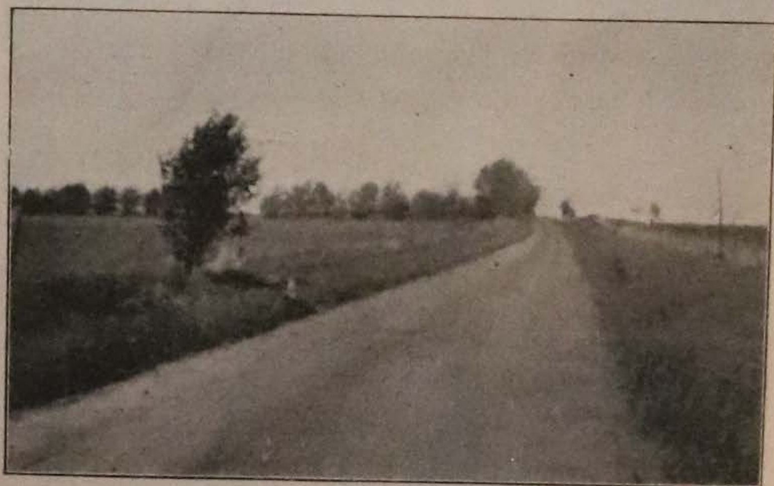
Fig. 20 GRAVEL ROAD SHOWING MAINTENANCE WITH A KING DRAG
