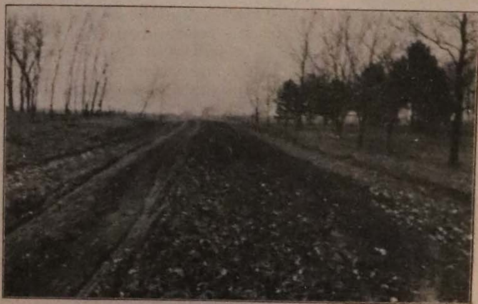
Fig 13—UNDRAINED ROAD IN SAC COUNTY, MARCH 28, 1905
