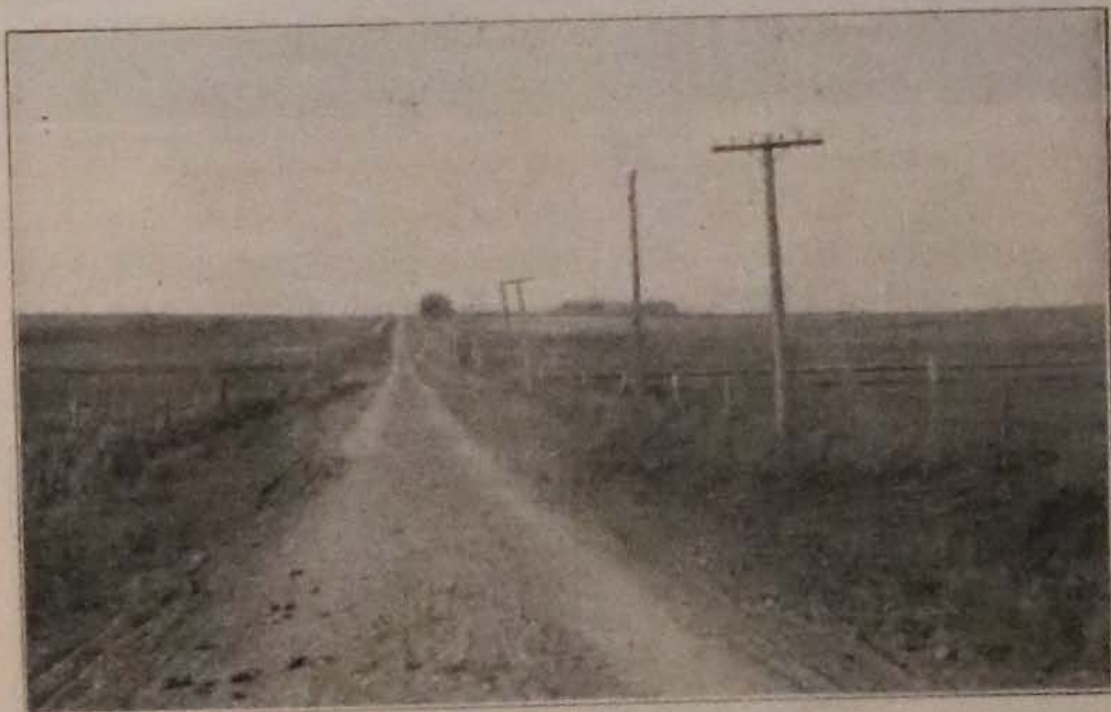
Fig. 18—ROAD IMPROPERLY DRAINED This stretch has been gravelled several times but gravel has disappeared each time.
