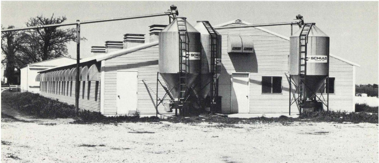
This modern farrowing-nursery structure with automated feed-handling is typical of “labor saving”.
