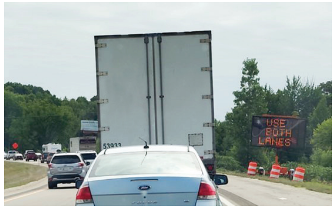
Roadside PCMS for lane merge management
