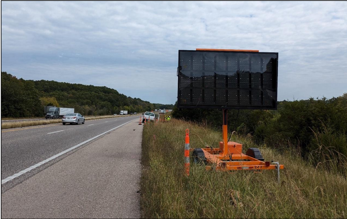
Figure 25. Roadside CMS for lane merge management
