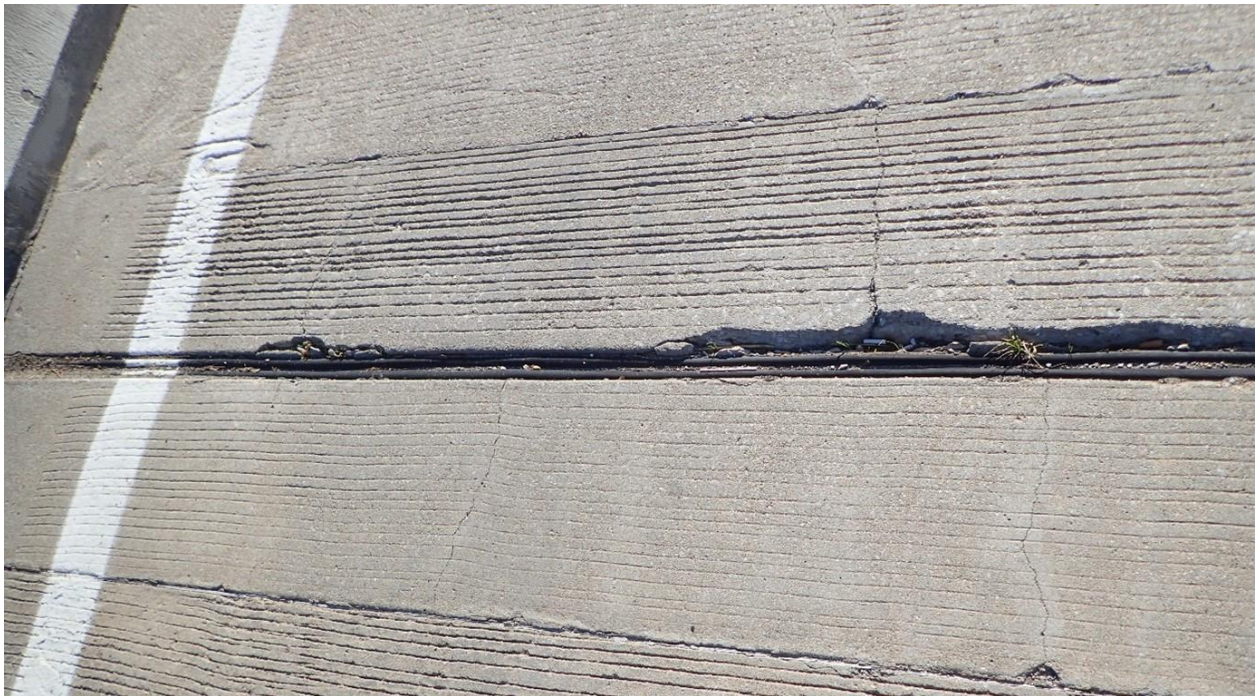
Figure 78. Compression seal joint in SR 46 Eastbound over East Fork White River
