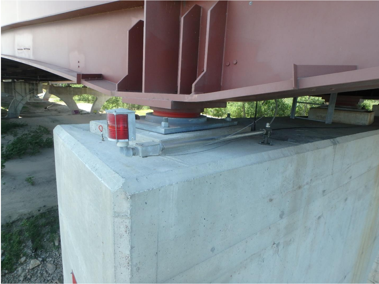
Figure 94. Disc Bearing on I-80 Westbound Bridge over Missouri River
