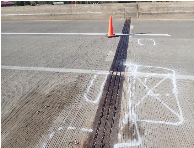
Figure 84. Modular joint on US 61 over Mississippi River
