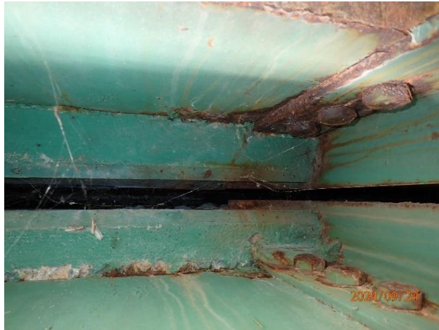
Figure 81. Underside of strip seal joint in US 61 over Mississippi River
