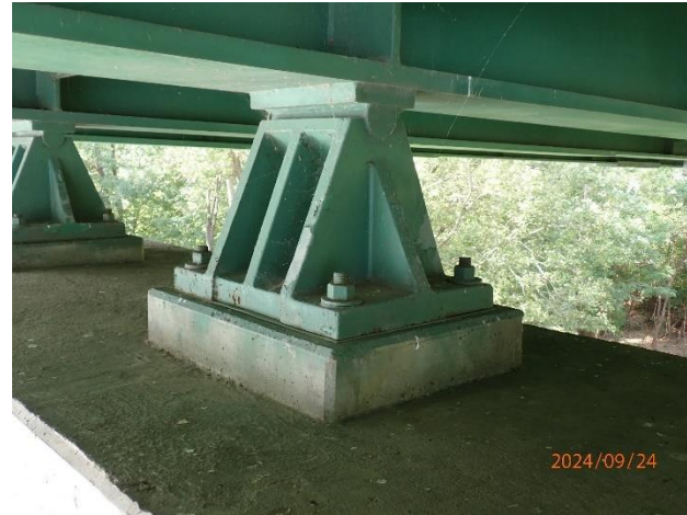
Figure 97. Fixed shoe on US 61 over Mississippi River
