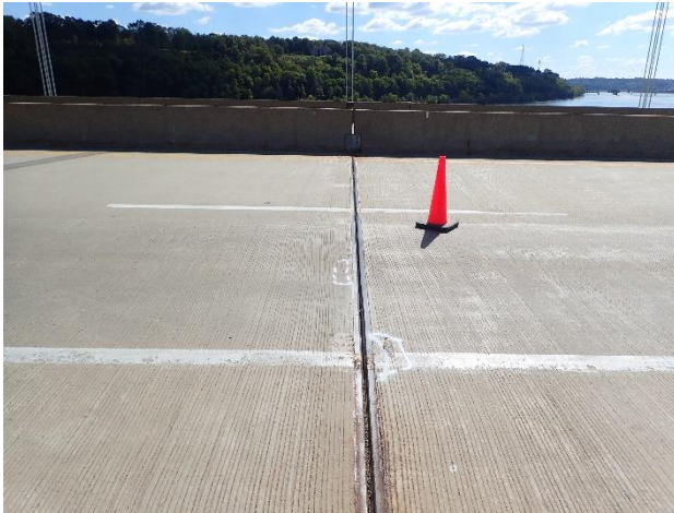
Figure 80. Strip seal joint in US 61 over Mississippi River
