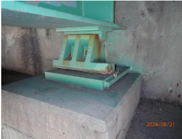
Figure 96. Rocker bearing on US 77 over Missouri River
