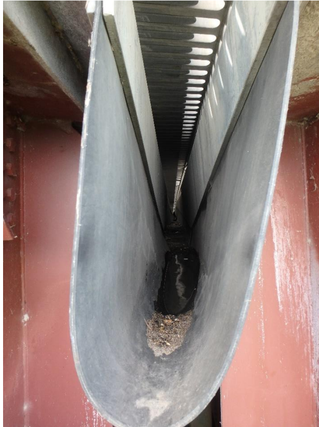
Figure 83. Neoprene trough beneath finger joint on I-80 Westbound over Missouri River
