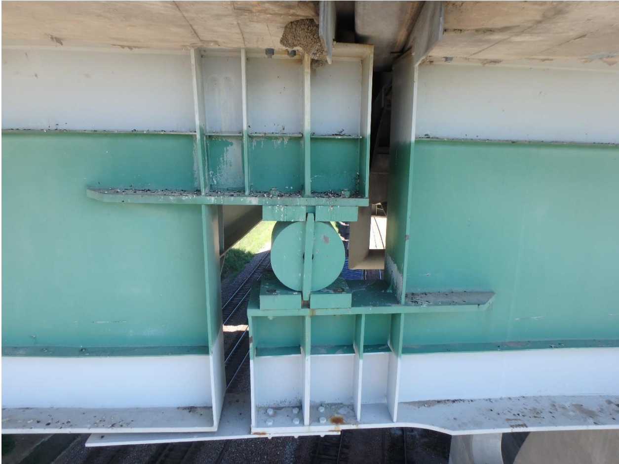
Figure 99. Roller hinge bearing on I-80 Eastbound over the Missouri River
