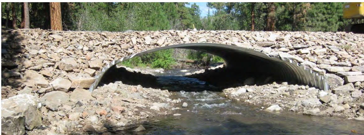
Forest Service bridge in Unity, Oregon.
