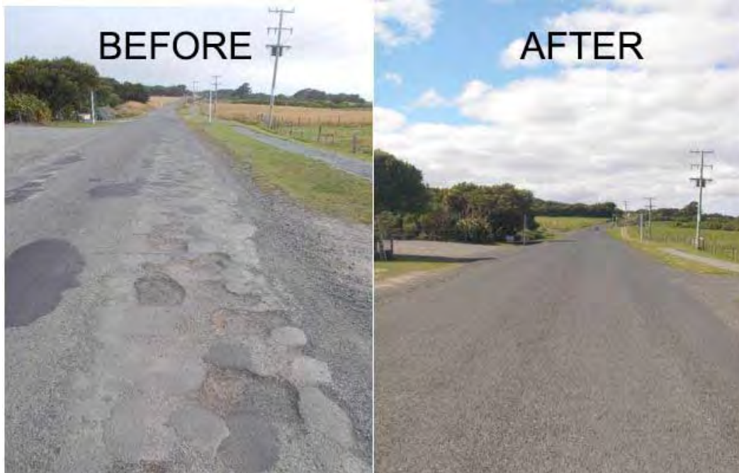
FIGURE 3 Photos of road reconstruction project on Chatham Island.
