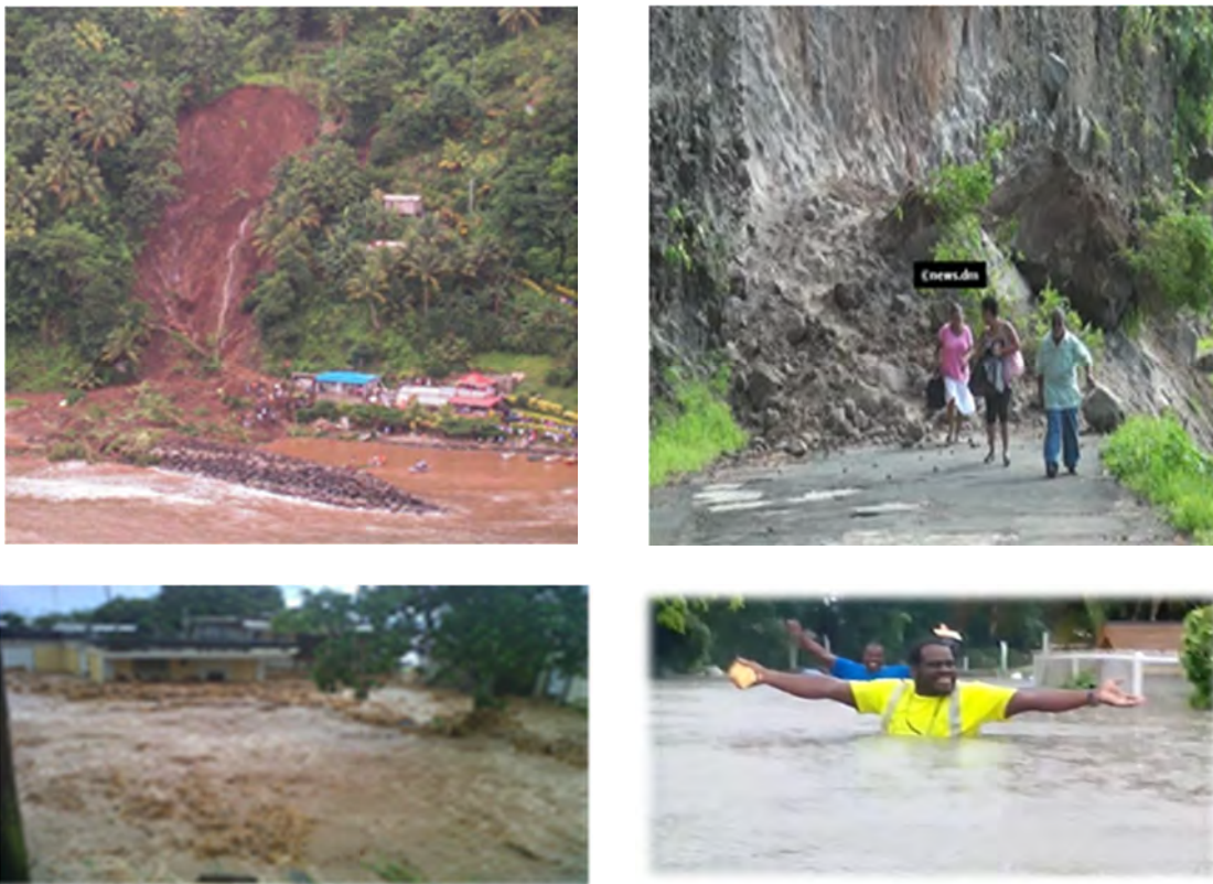
FIGURE 1 Impact of ongoing climate changes and related heavy rainfall and flooding events on roads, structures, and local endangered species. The four photos present Dominica's typical erosion, landslide failures, and flooding attributed to weakened vegetation as a result of rising ambient temperature and prolonged drought periods.
