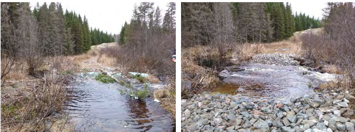
FIGURE 2 Site 101+100 before and after construction work, November 2018.
