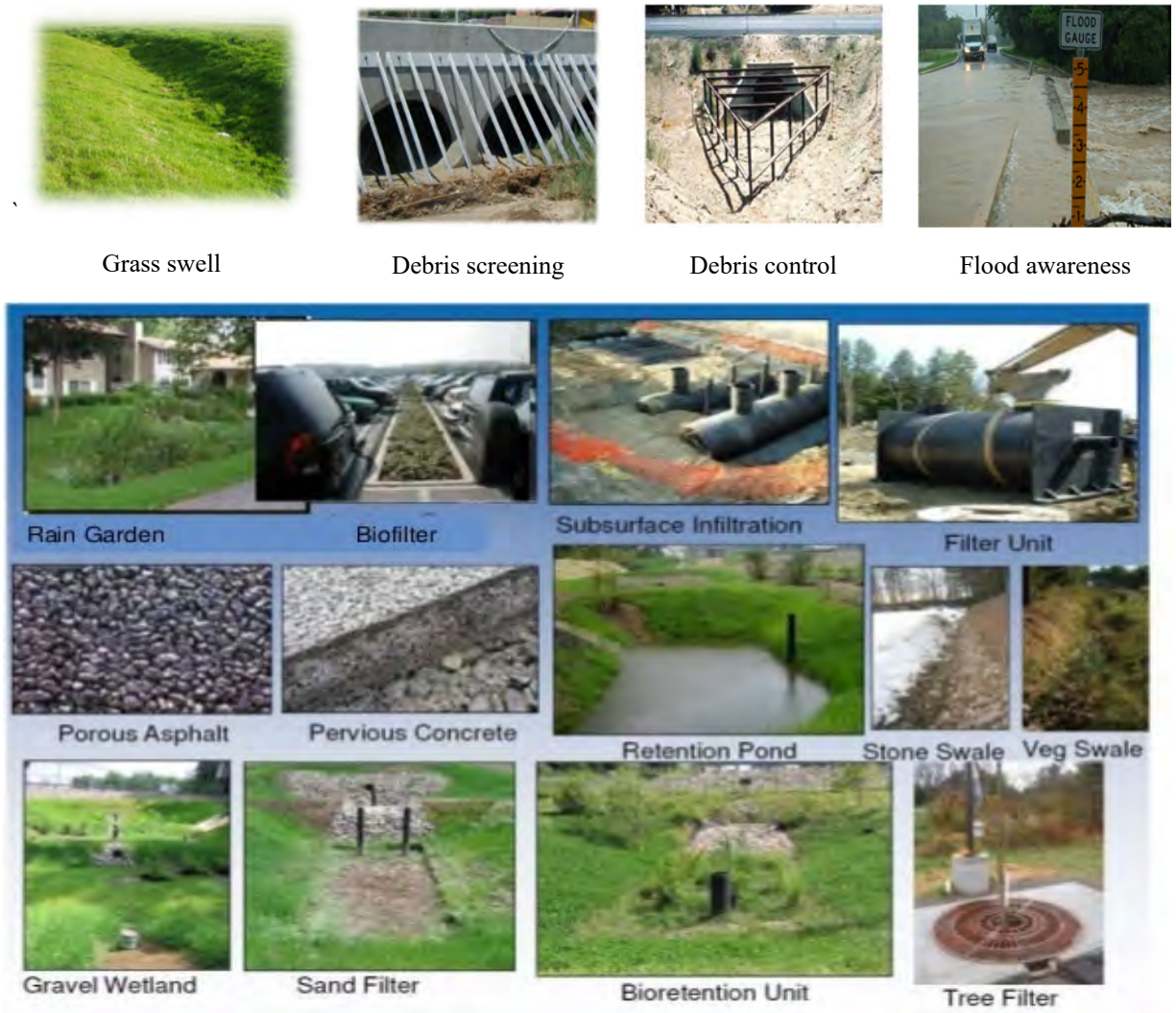
FIGURE 3 Cost-effective stormwater management tools, including debris control elements given in the two-upper-center photos and other stormwater management and sediment control and retention facilities used to avert environmental degradation of threatened marine species in the Caribbean coastal areas.
