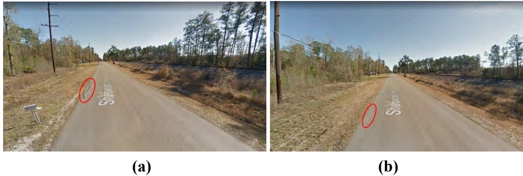
FIGURE 7 Google map street images of Sherwood Drive, looking towards Tram Road in Beaumont, captured in January 2013: (a) sealed cracks and (b) developing cracks. (Map data © 2018 Google.)
