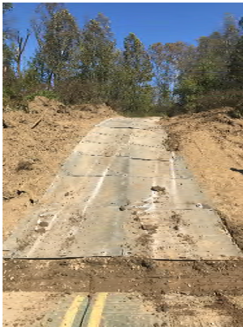
FIGURE 8 Damage to ACE Mat from bulldozer, Fort Knox test site.
