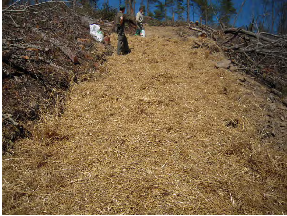
FIGURE 6 Students can examine and monitor a variety of erosion control techniques used on roads and skid trails such as this seed and mulch treatment used on a bladed skid trail.
