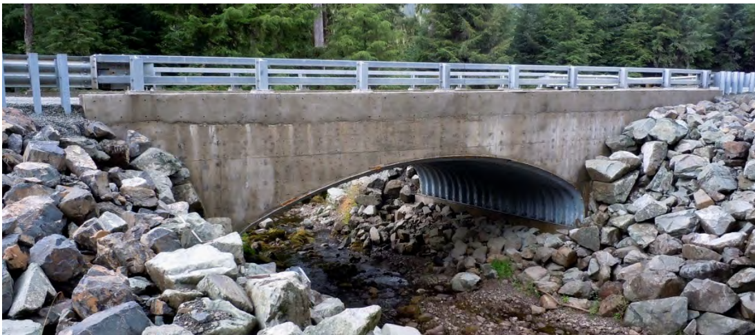
Bridge built by tribal forces near Craig, Arkansas.
