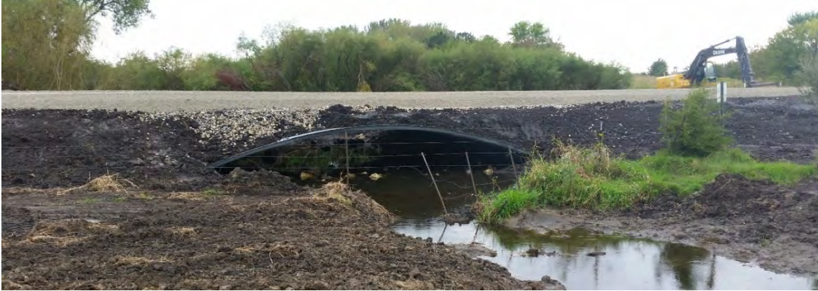
Replacement for timber bridge on farm road in Buchanan County, Iowa.
