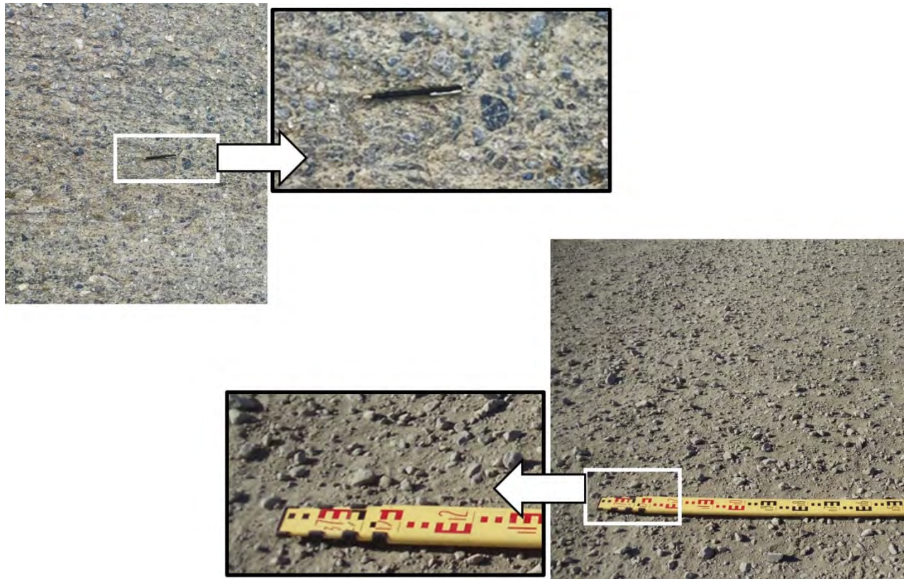
FIGURE 6 Close up of a premium pavement (upper left) after three rainy seasons, compared to an untreated pavement (lower right) with considerable unbound material because of loss of fines after rain.
