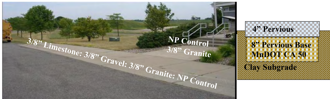
FIGURE 3 Pervious concrete MnROAD sidewalk with cross-section ( right ).
