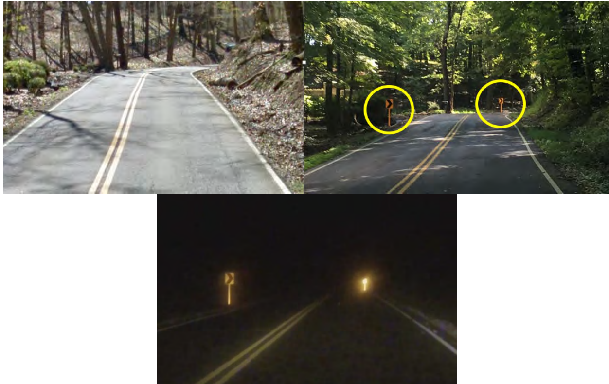
FIGURE 2 Before (upper left) and after (upper right, lower center) images of the same signage installation.
