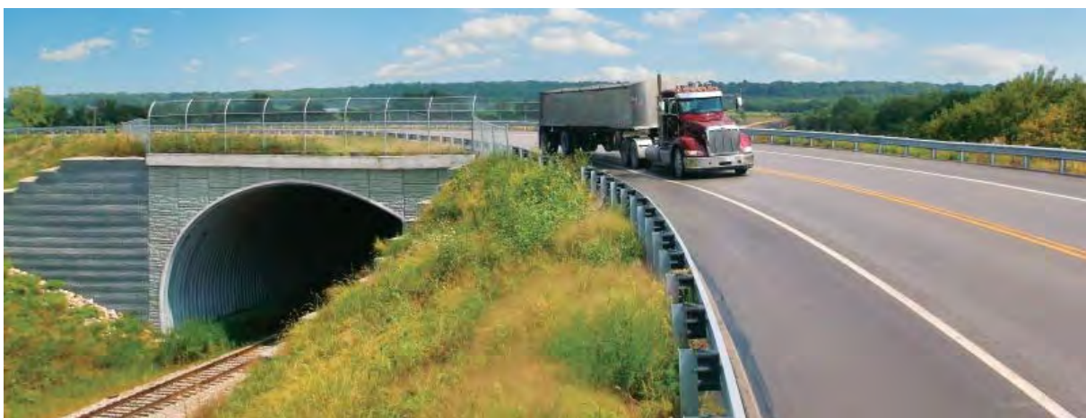
Grade separation—county road over dual track rail crossing near LaCygne, Kansas.
