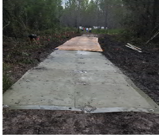
FIGURE 2 Apalachicola National Forest ACE Mat installation.
