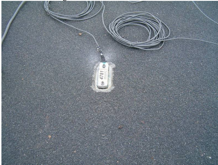
Figure 17. Top of Deck Test Instrumentation, individual strain gage.
