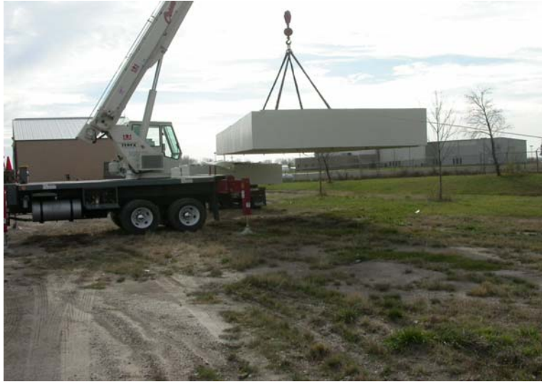
Figure 11. Unloading of individual deck panels.
