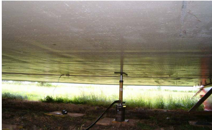
Figure 14. Hydraulic Jack.
