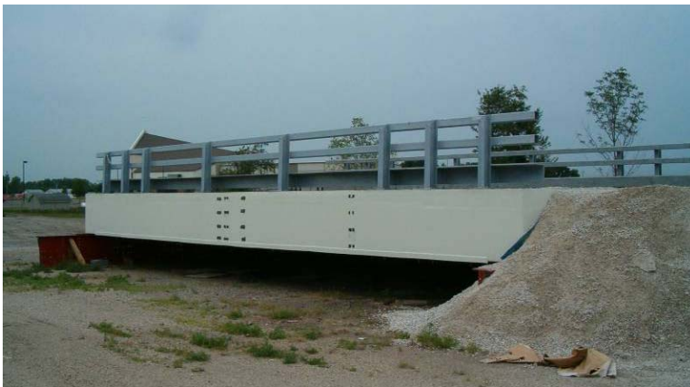
Figure 13. FRP Bypass Bridge with guardrail installed.
