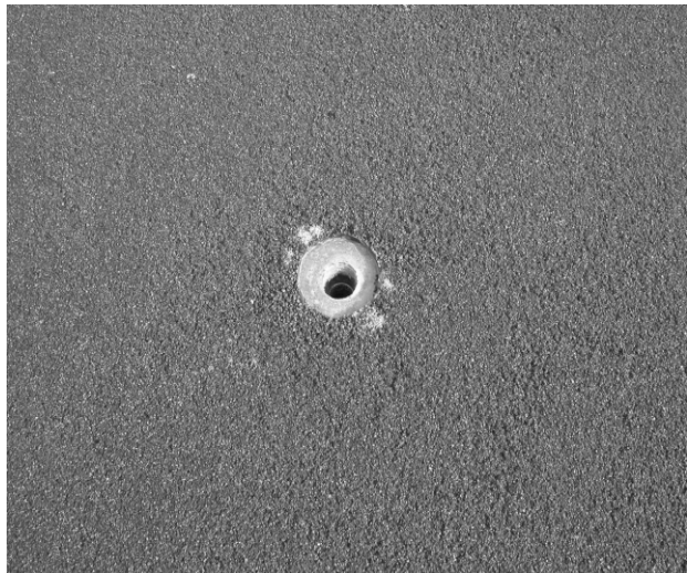
Figure 8. Threaded insert for installation of lifting lugs
