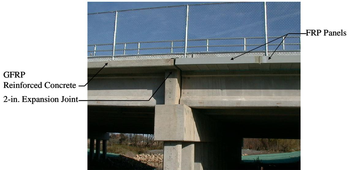
**Figure 7. Expansion Joint Detail**
