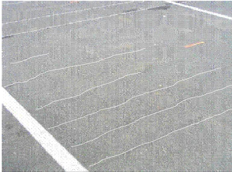
**Figure 55. Transverse Cracks in South Traffic**
