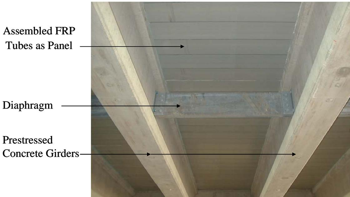
**Figure 13. FRP Deck - Bottom Surface**
