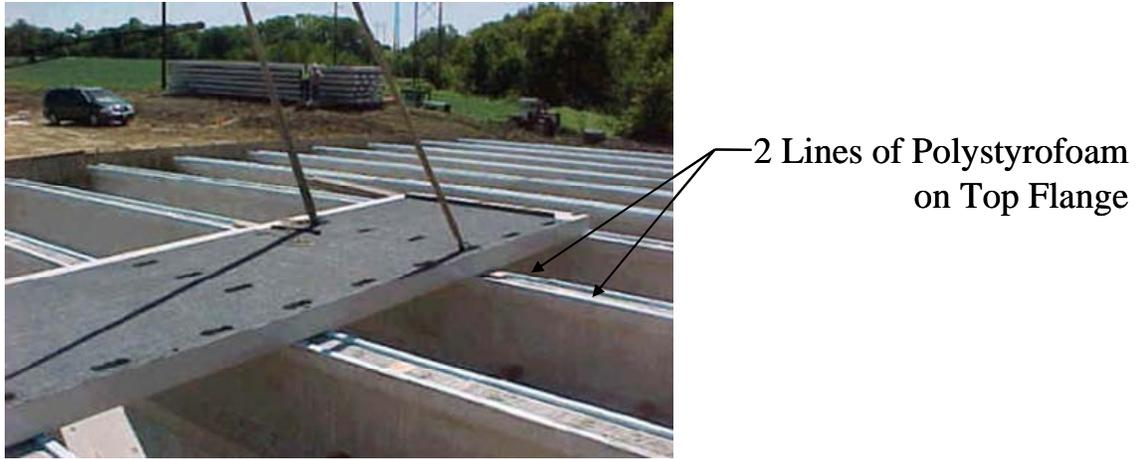
**Figure 10. Installation of the FRP Panel Deck**
