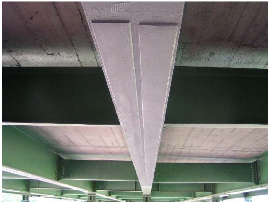
(c) Girder 4 in the east end span
