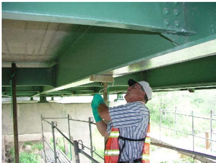
Figure 14. Applying FRS 1000 Primer to bottom girder flange.
