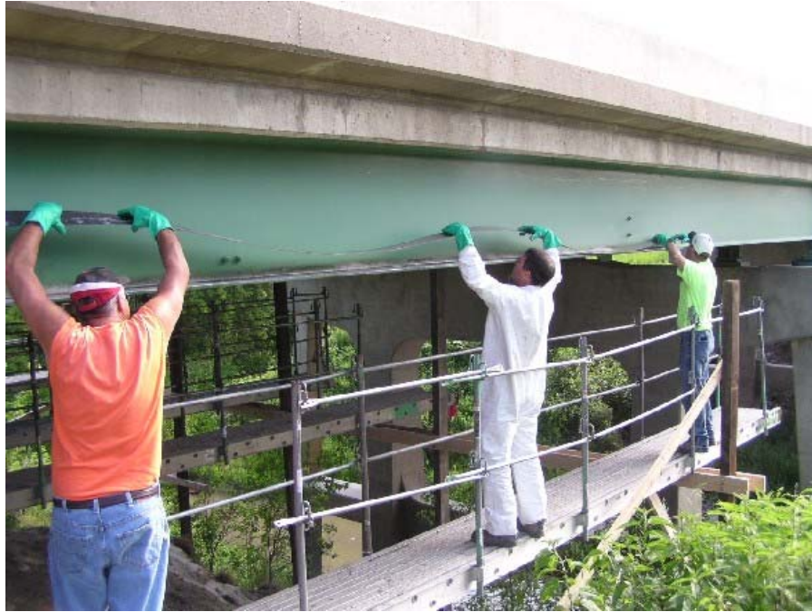
Figure 18. Placement of CFRP plate on top of Girder 6 bottom flange.
