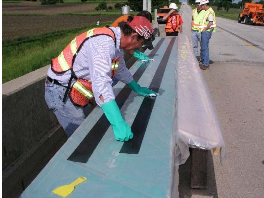
Figure 13. Cleaning the CFRP plate bonding surface.
