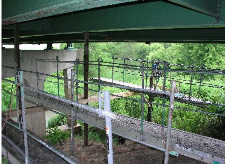
Figure 9. Temporary work scaffolding.
