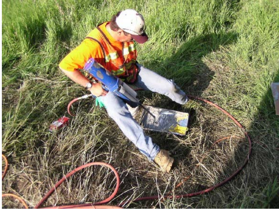
Figure 15. Preparation of ECS 104 structural epoxy (mixing with a compressed air gun).
