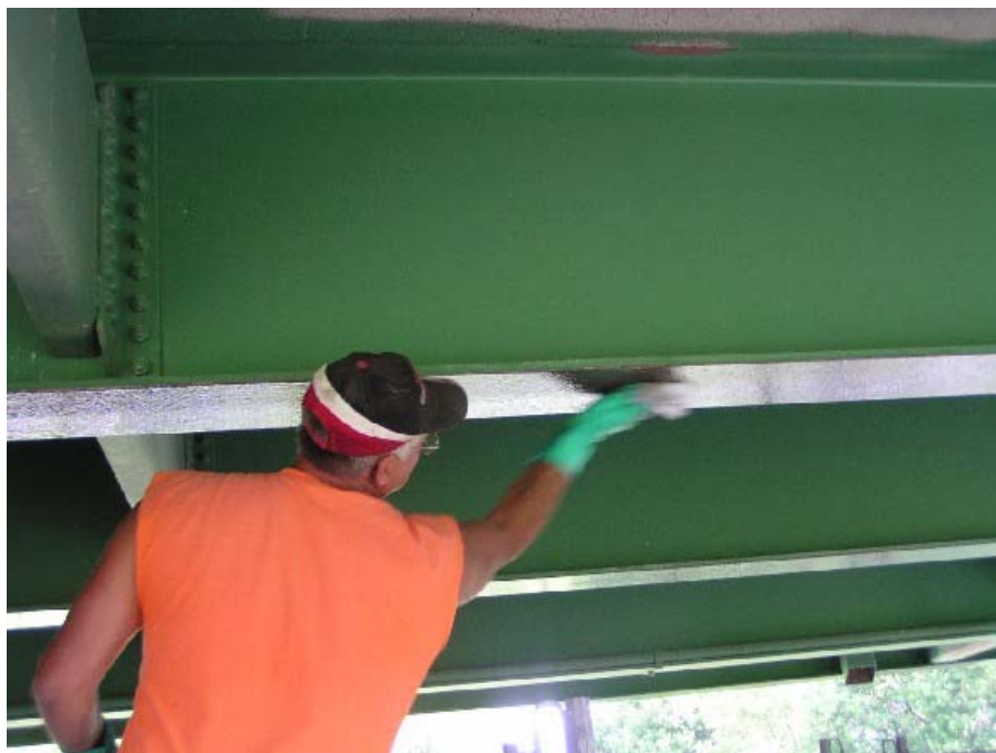
Figure 12. Cleaning the girder surface after sandblasting.
