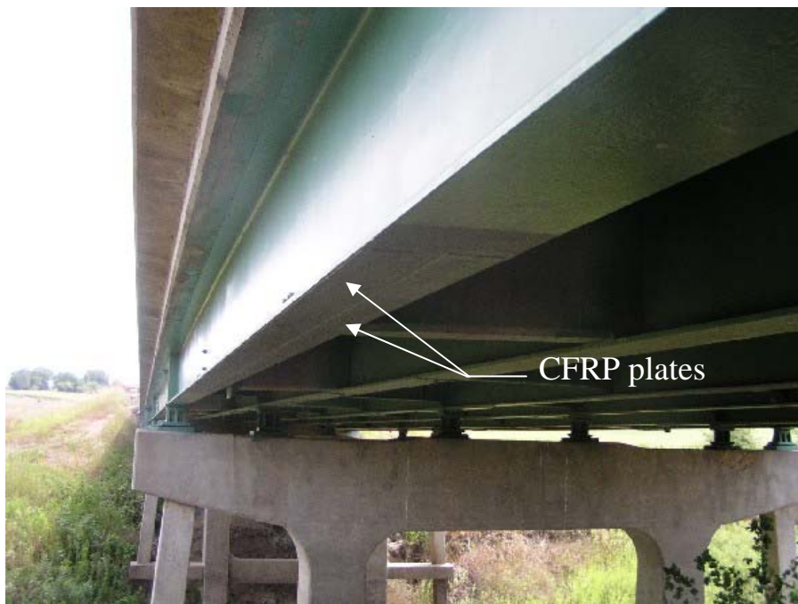
(a) Girder 1 in the west end span
