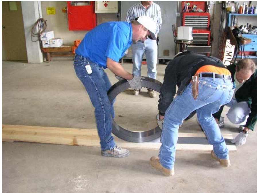
Figure 3. CFRP plates being unrolled.
