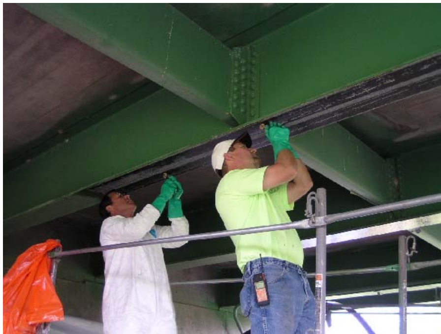
Figure 19. Removal of excess air by applying pressure with a roller.
