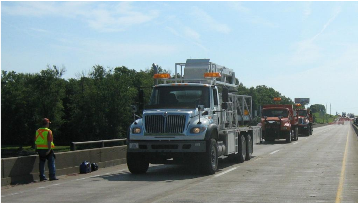
Figure 15. Load Case 1 (Iowa DOT snooper, Truck 2 and Truck 1 back-to-back-to-back in middle lane). Trucks are separated by approximately 20 ft and are in the north lane.
