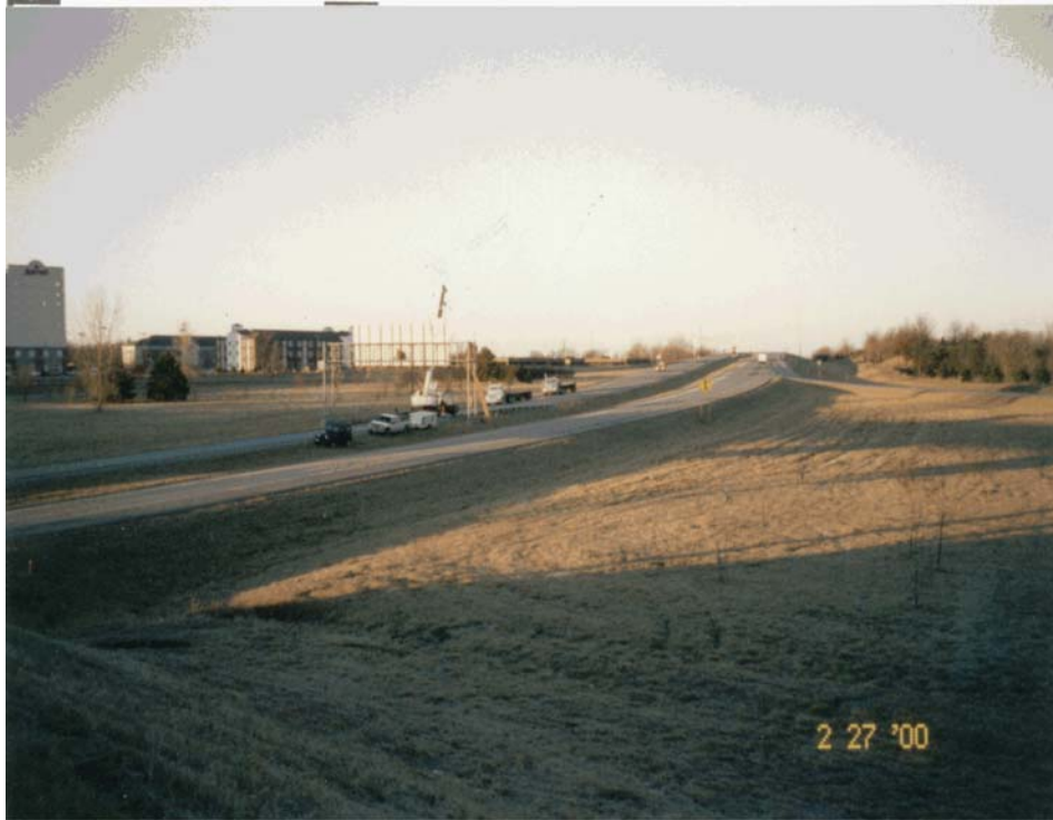
a. Overview of the Sign Truss Site
