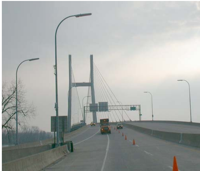
Figure 3. Typical photograph of bridge (looking to the East).
