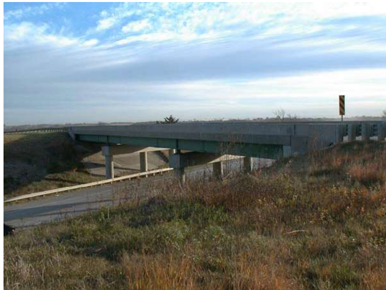
Figure 3.1. Photograph of test bridge looking northeast.
