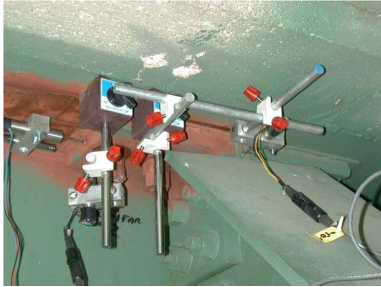
Figure 5.10. Photograph of displacement transducers at retrofit.
