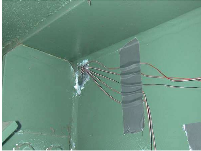
a. Close-up of typical gradient gage.
