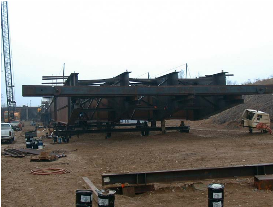
Figure 3.11. Rear of launching tail showing transverse tugger beam.
