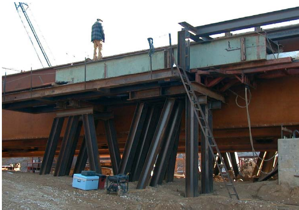
Figure 3.9. Gantry assembly supporting the hydraulic cylinder.
