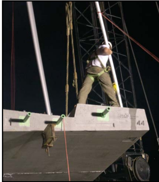
Figure 2. Installation of instrumented hanger rod in 44 th Street Bridge
