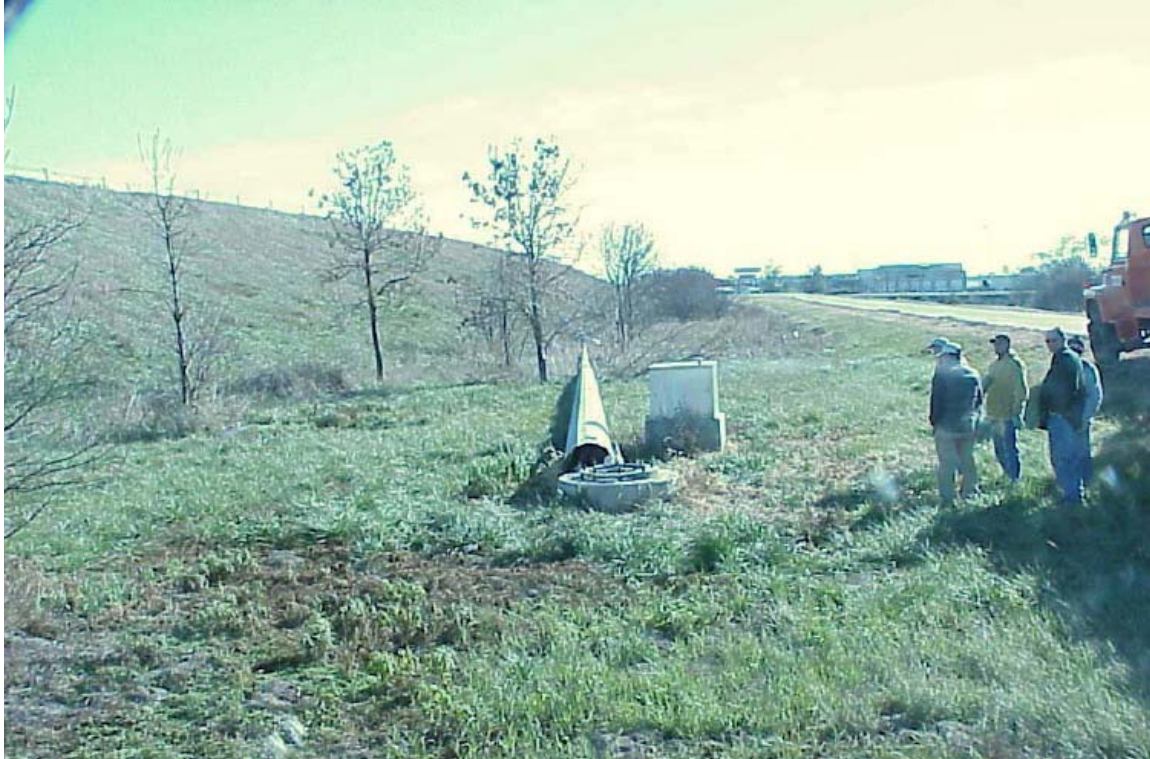
Figure 1-1. A collapsed high-mast light pole along I29 near Sioux City in 2003
