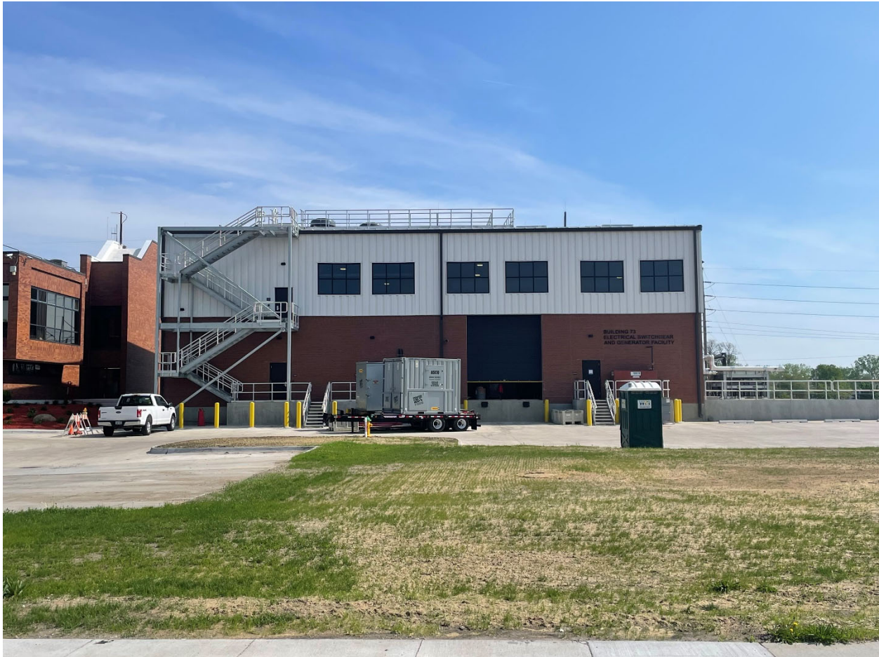
Figure 1: New Standby Power and Electrical Service Building
