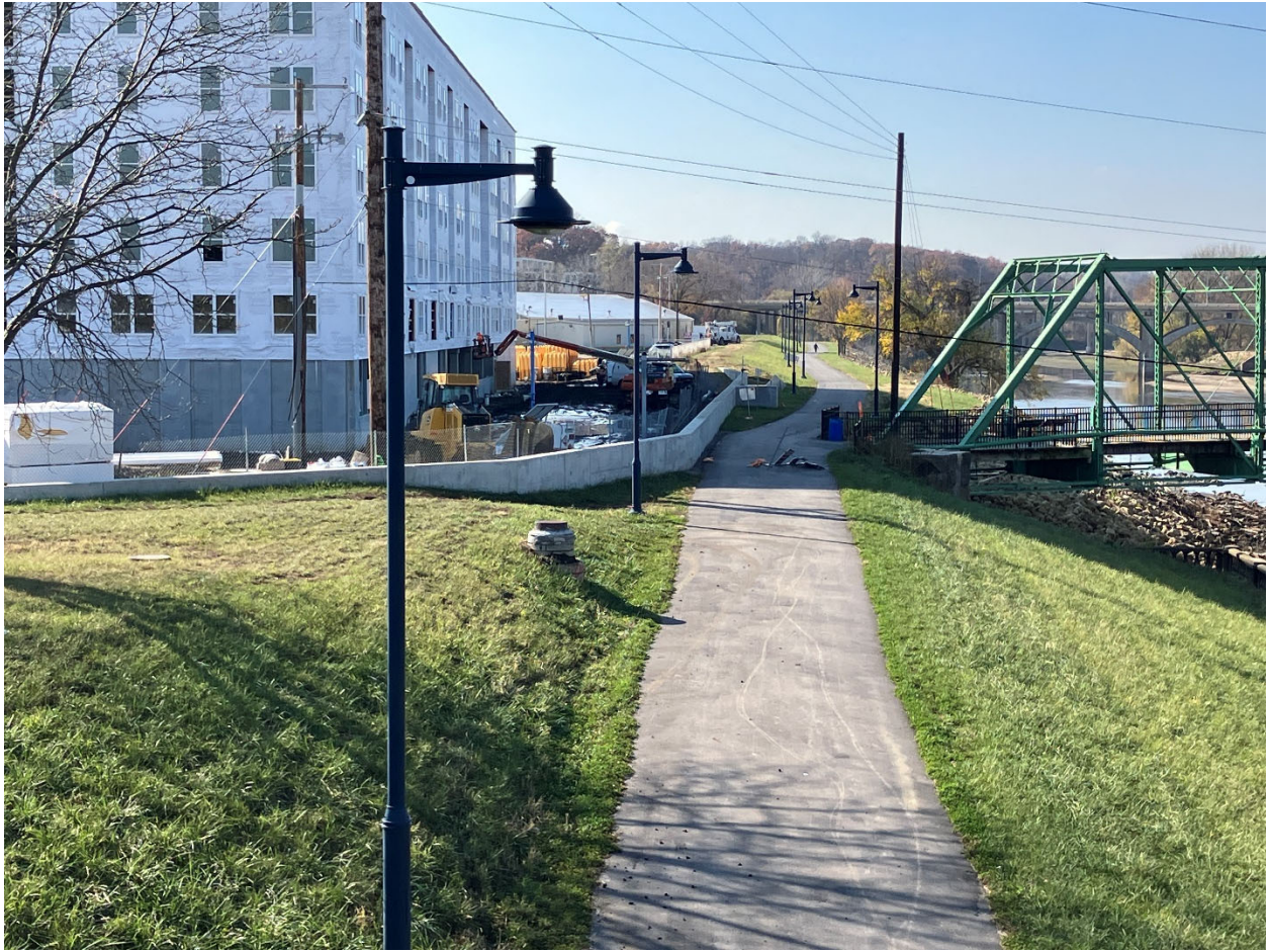
DSM Levee Alt Phase B, SW 3 rd Street - SW 7 th Street, south side floodwall
