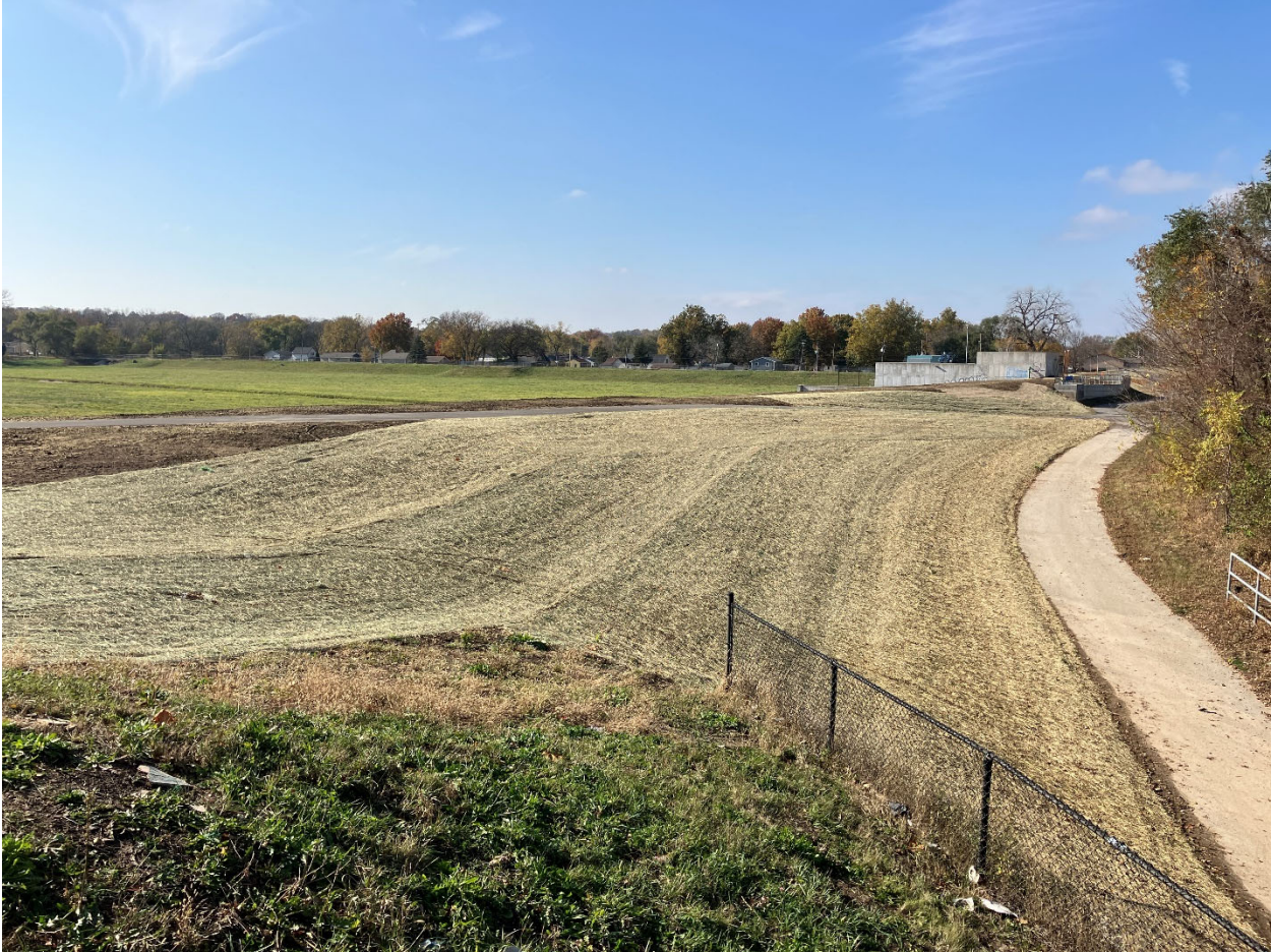
DSM Levee Alt Phase C, south side of Des Moines River between SE 14 th Street & Jackson Pump Station
