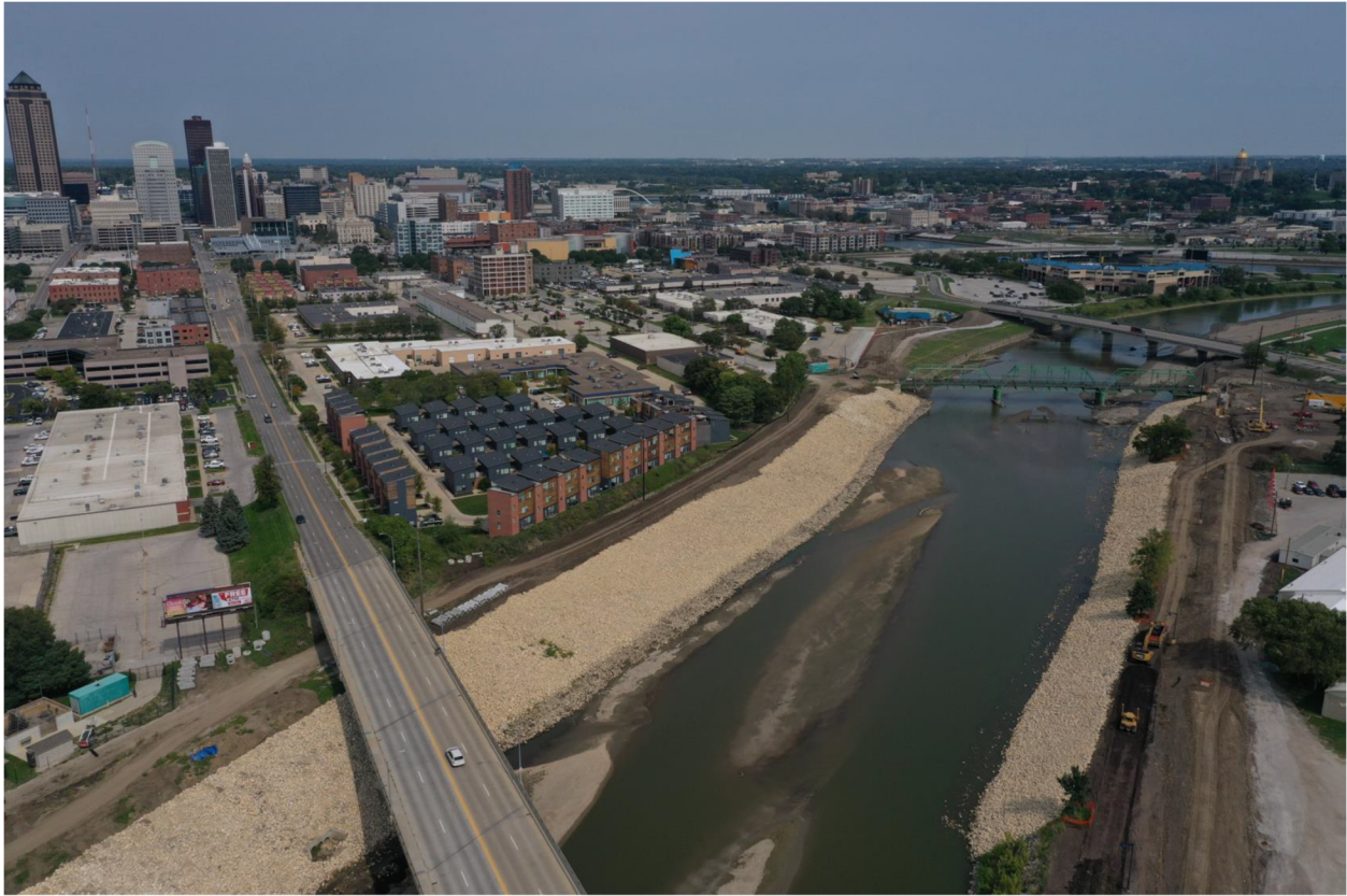
Photo from Parks and Recreation drone above SW 7 th Street bridge looking down stream
