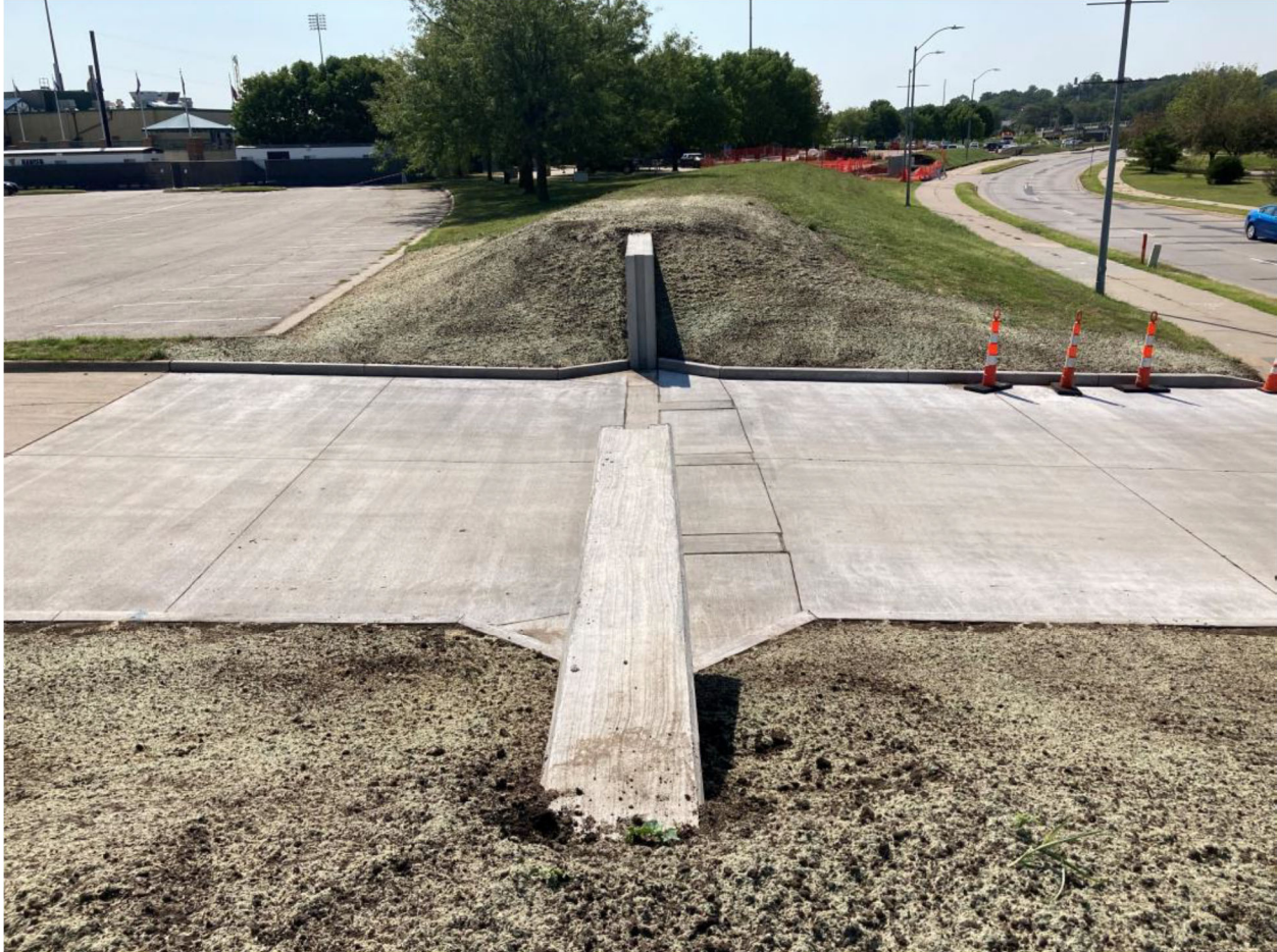
New stop log closure installed as part of Phase A of the Levee Alterations at the parking lot access at Principal Park.
