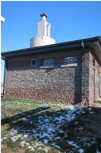
New water treatment plant building with aerator
