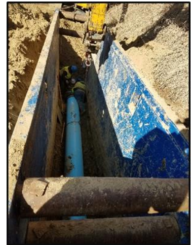
Water main installation using open trench construction (photos were provided by the system)
