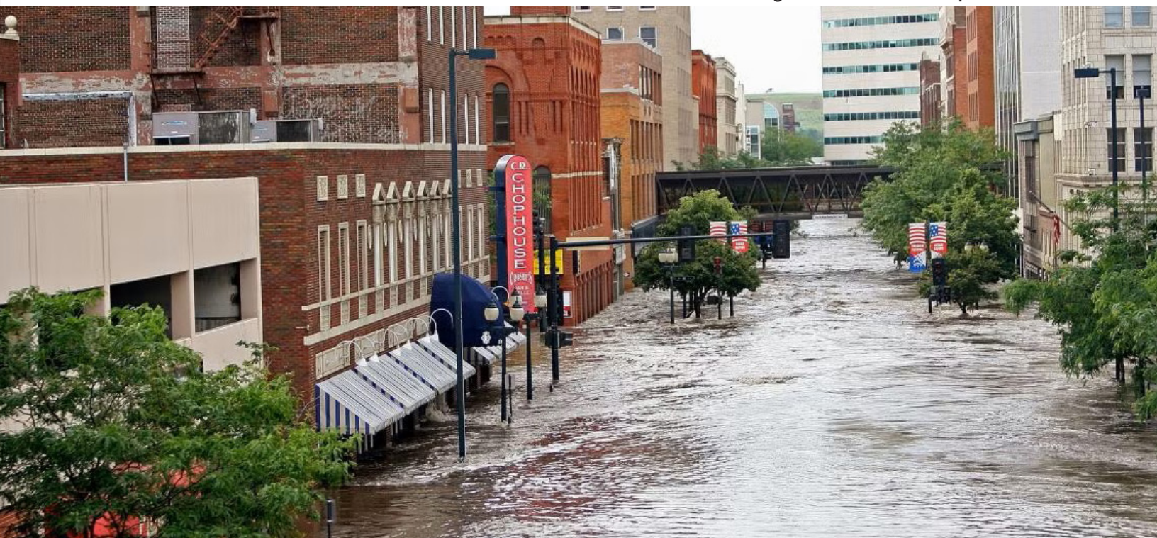
Flooding in downtown Cedar Rapids in June 2008
