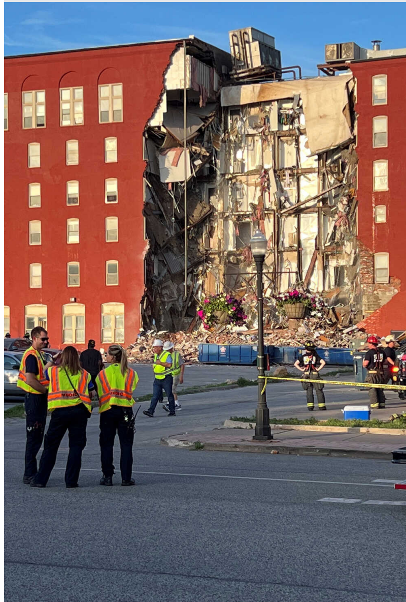
Partial apartment building collapse in Davenport in May 2023
