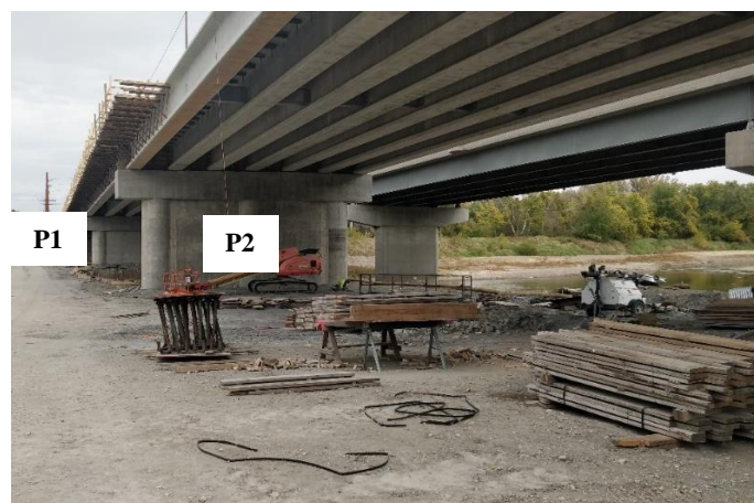
Figure 30. Girders and piers constructed over the shafts, Polk County
