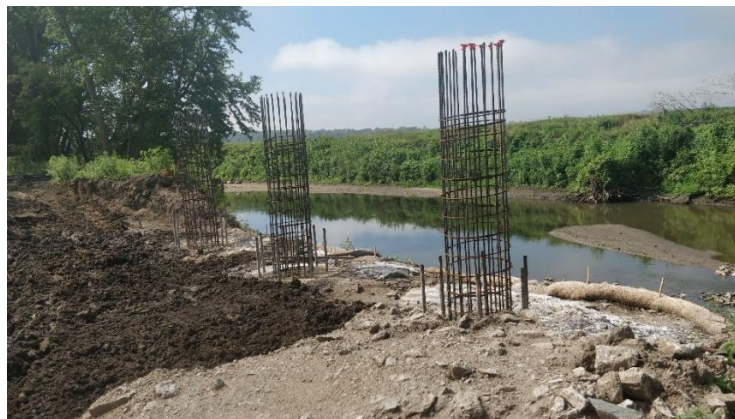
Figure 27. Completed drilled shaft construction, Polk County
