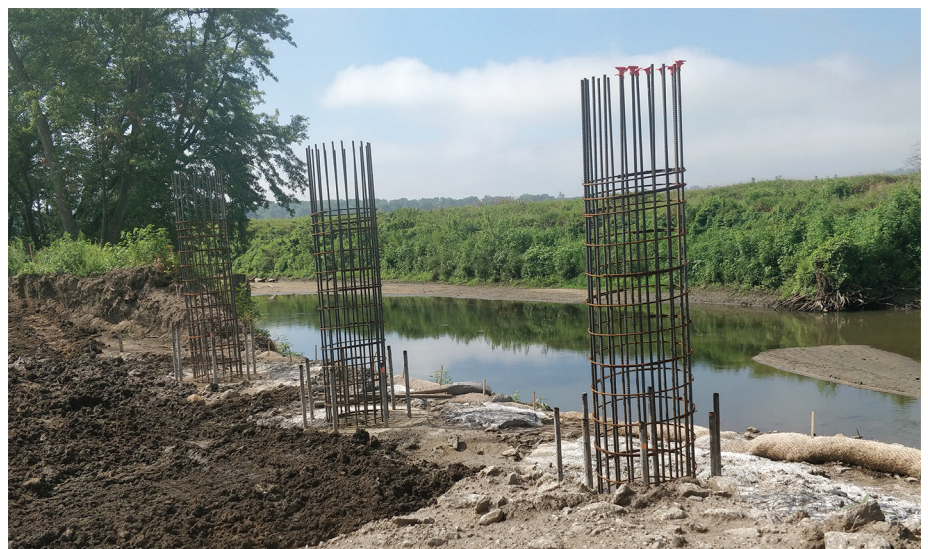
Completed construction of drilled shafts
