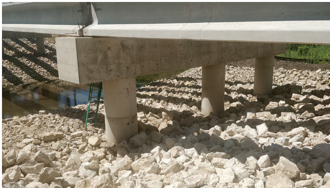
Drilled shafts after placement of pier caps and girders
