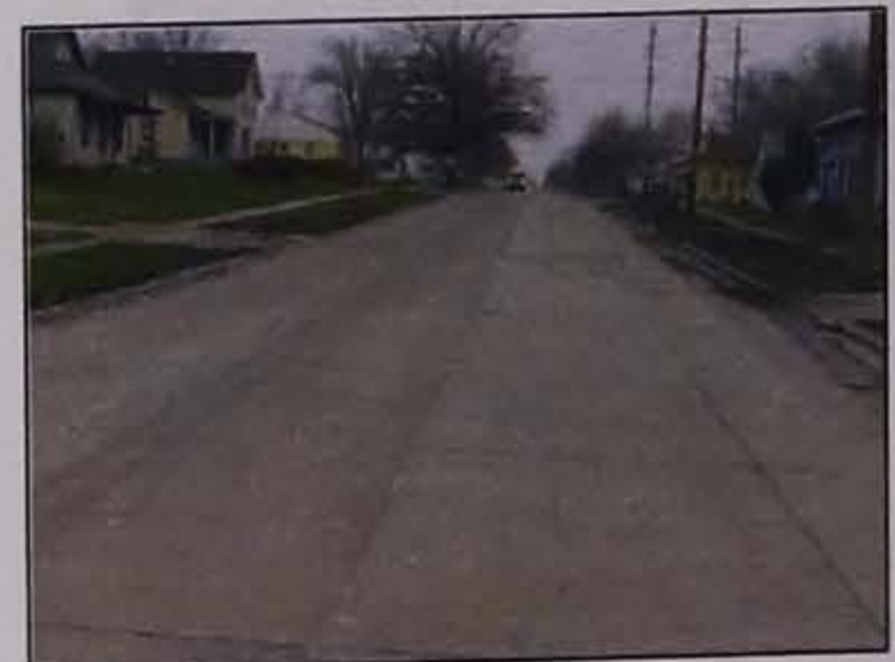
Completed Jointing Pattern
