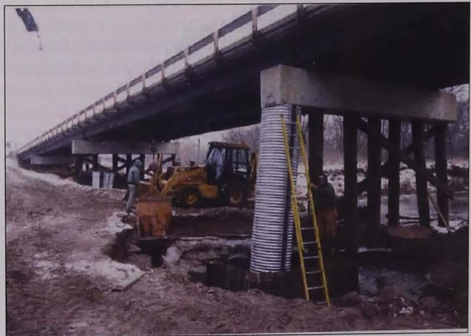
Jacketing of Deteriorated Timber Piles
