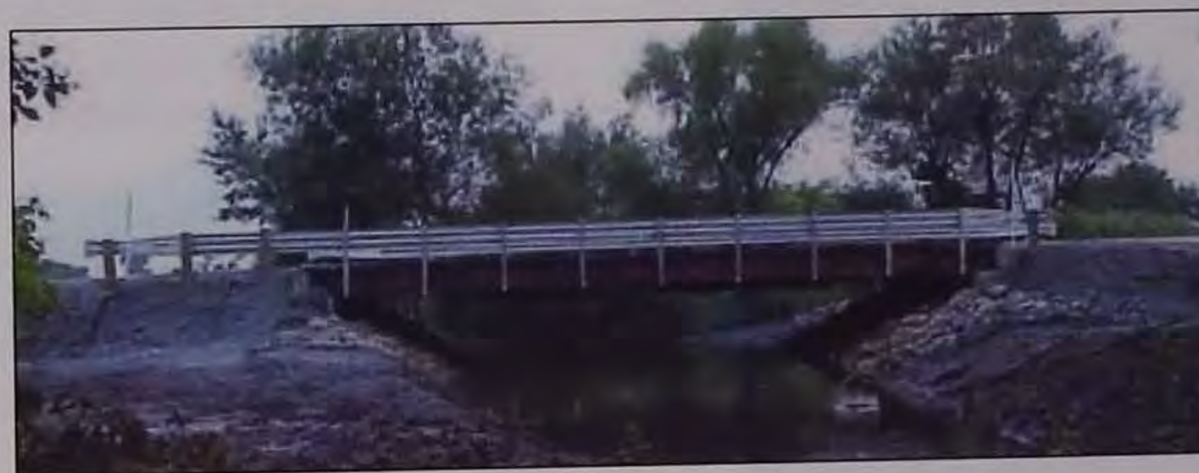
Finished Buchanan County RRFC Bridge
