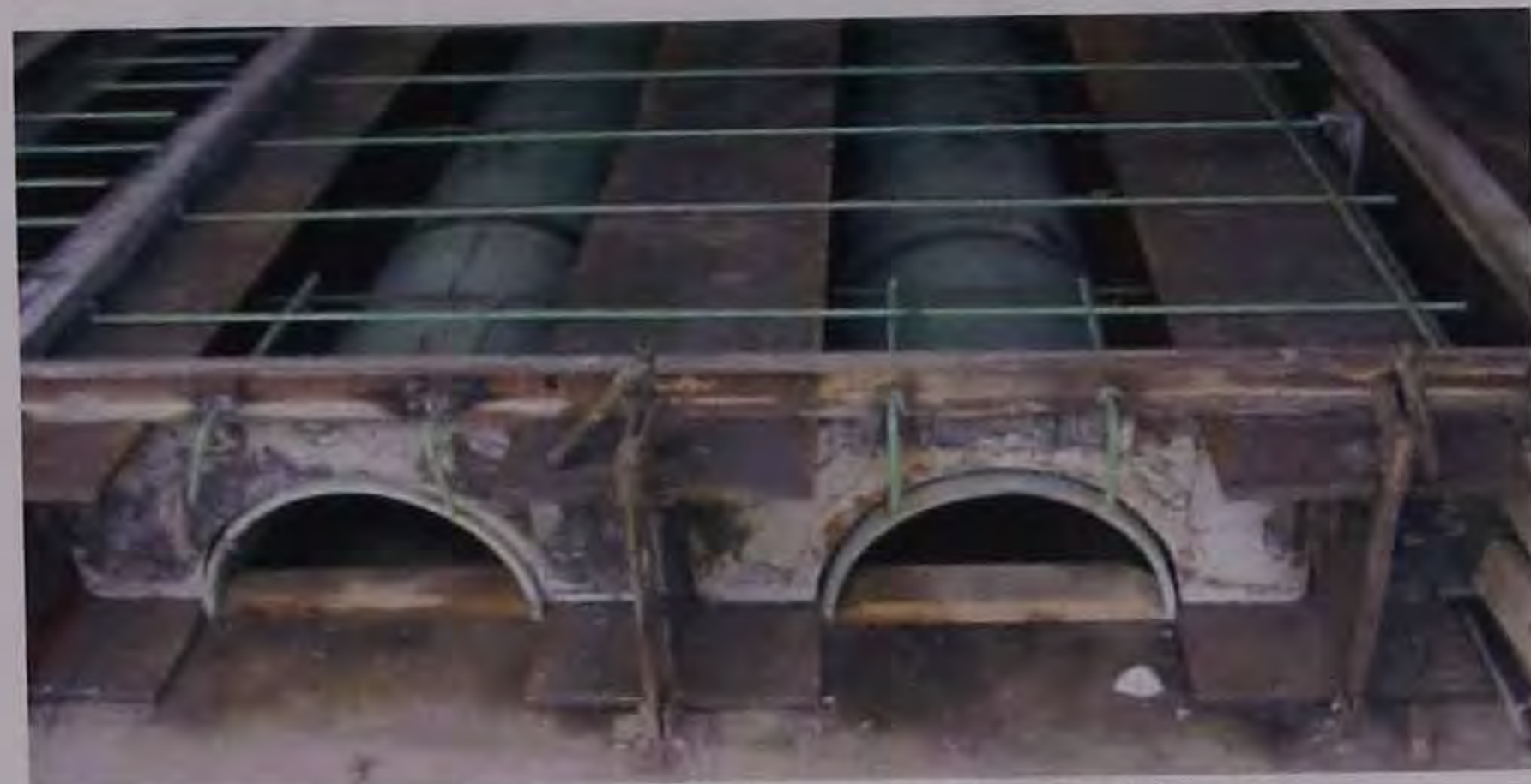
Transverse arches between the steel beams.
