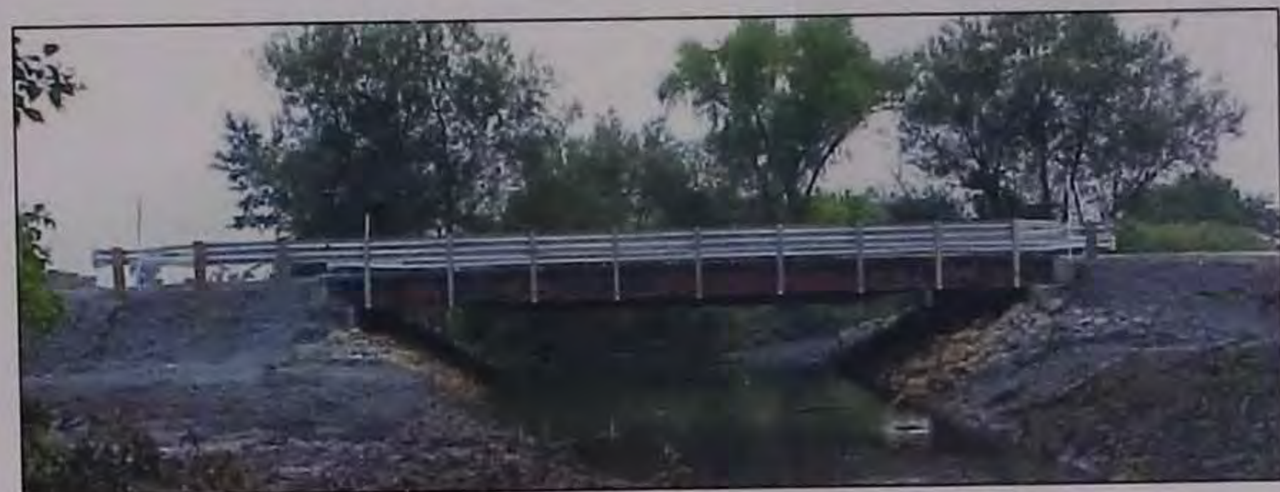
Finished Buchanan County RRFC Bridge
