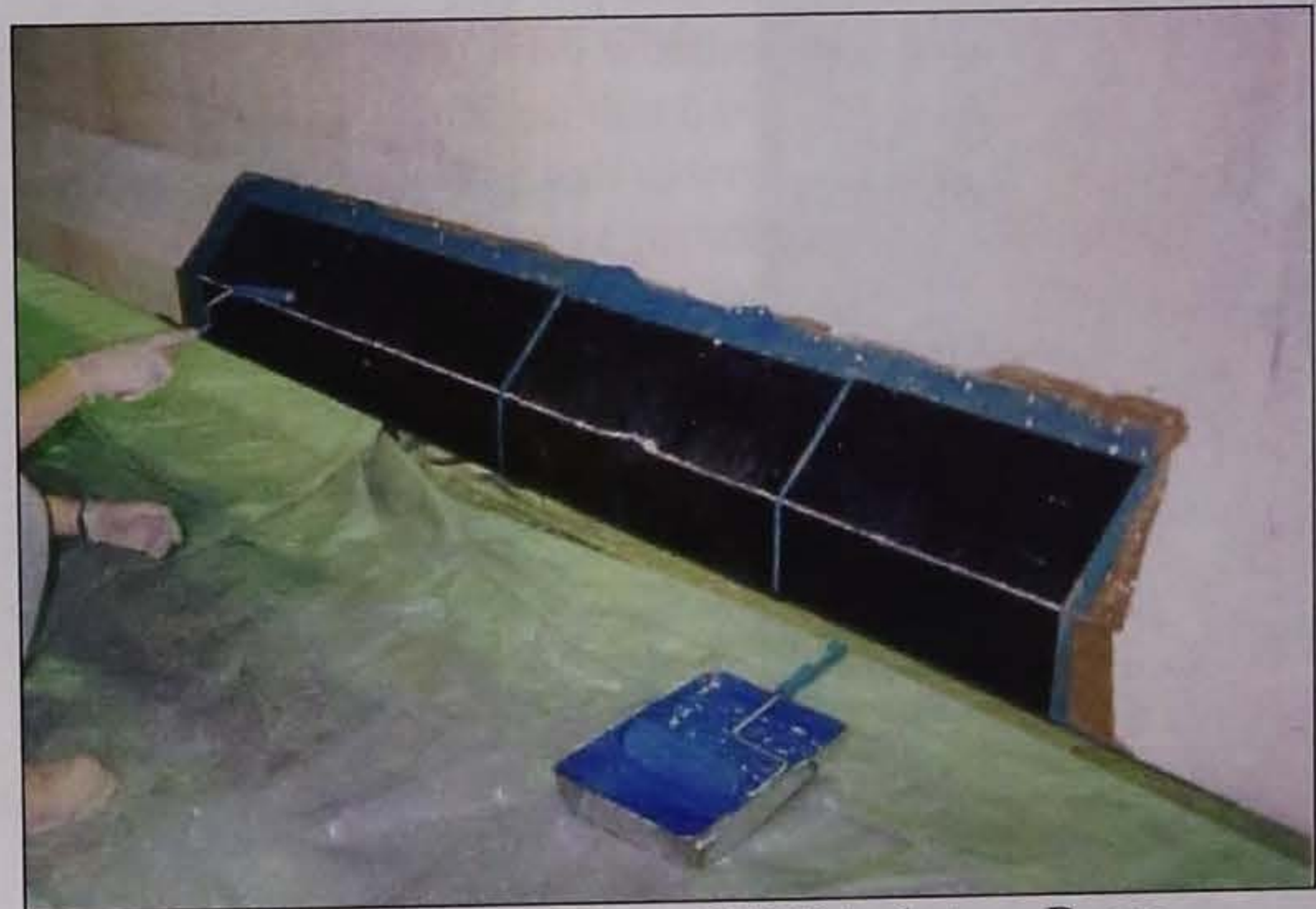
Installation of transverse CFRP jacket on Beam
