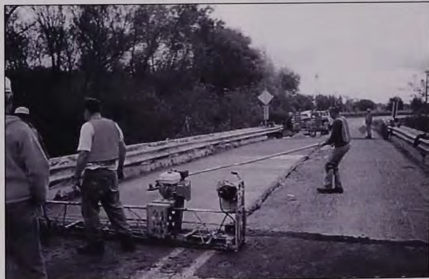
PCC Placement on the Independence Bridge
