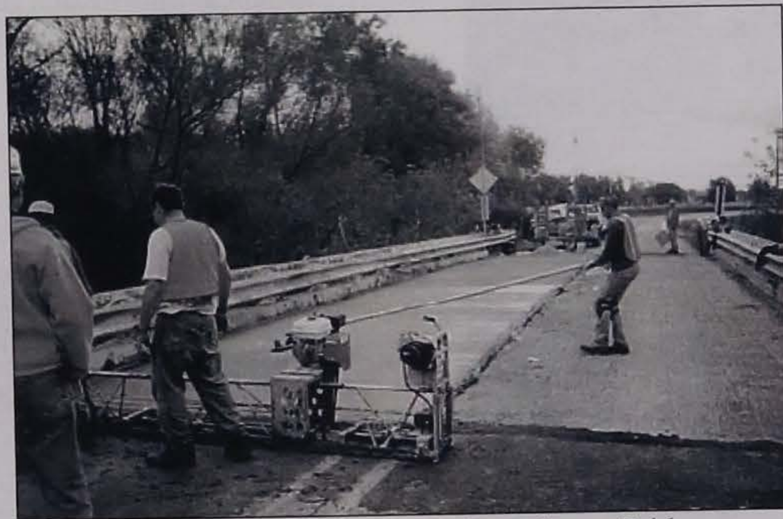
PCC Placement on the Independence Bridge
