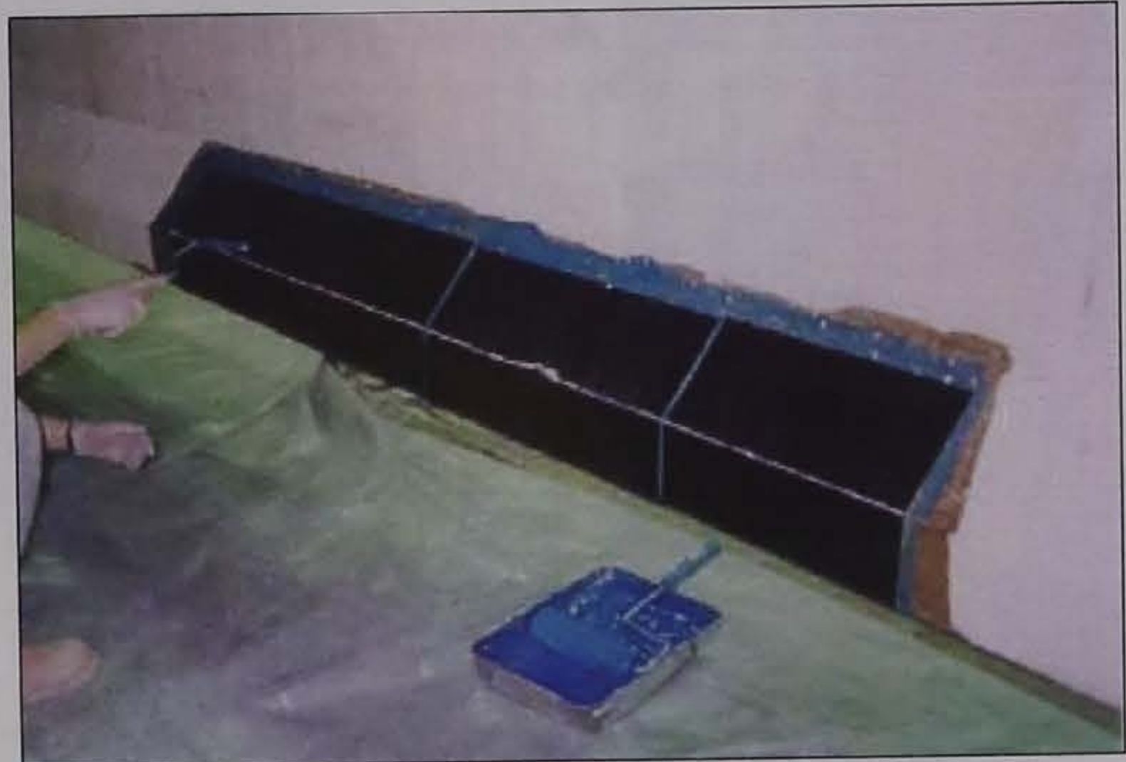
Installation of transverse CFRP jacket on Beam
