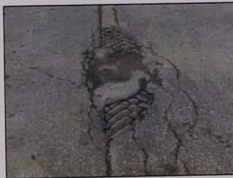
Asphalt Surface with Exposed Brick
