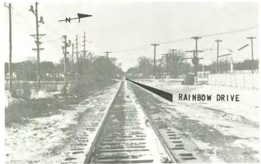
Photo No. 14. C.R.I.&P. Railroad at Rainbow Drive.
