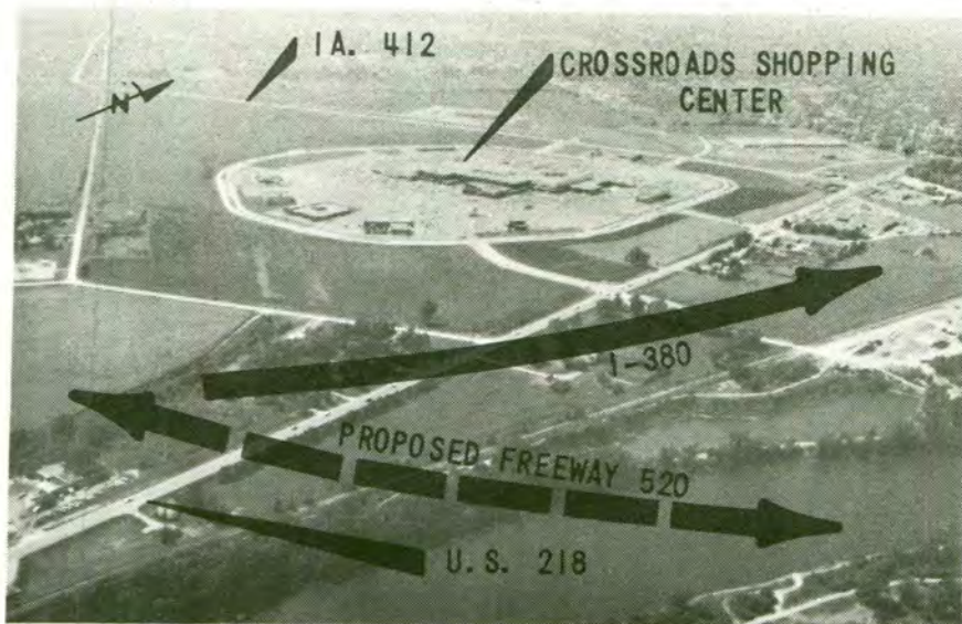
Photo No. 1. Beginning of Project.
