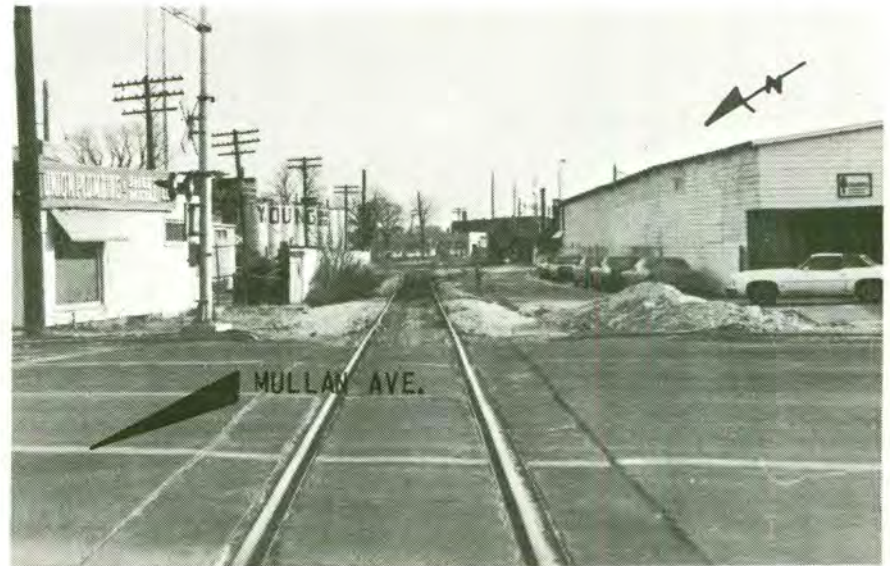
Photo No. 10. C.R.I.&P. Railroad at Mullan Avenue.
