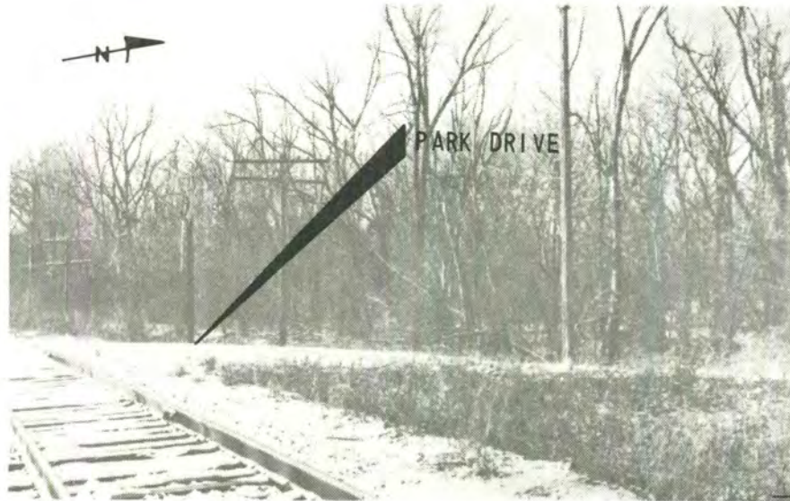
Photo No. 15. Location Near Park Drive, Alternatives A and B.
