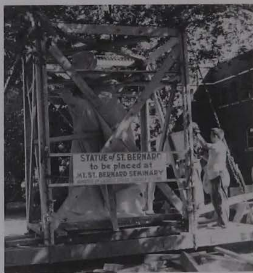
LOADING ON TRUCK FOR TRANSPORT TO DUBUQUE. CPP
