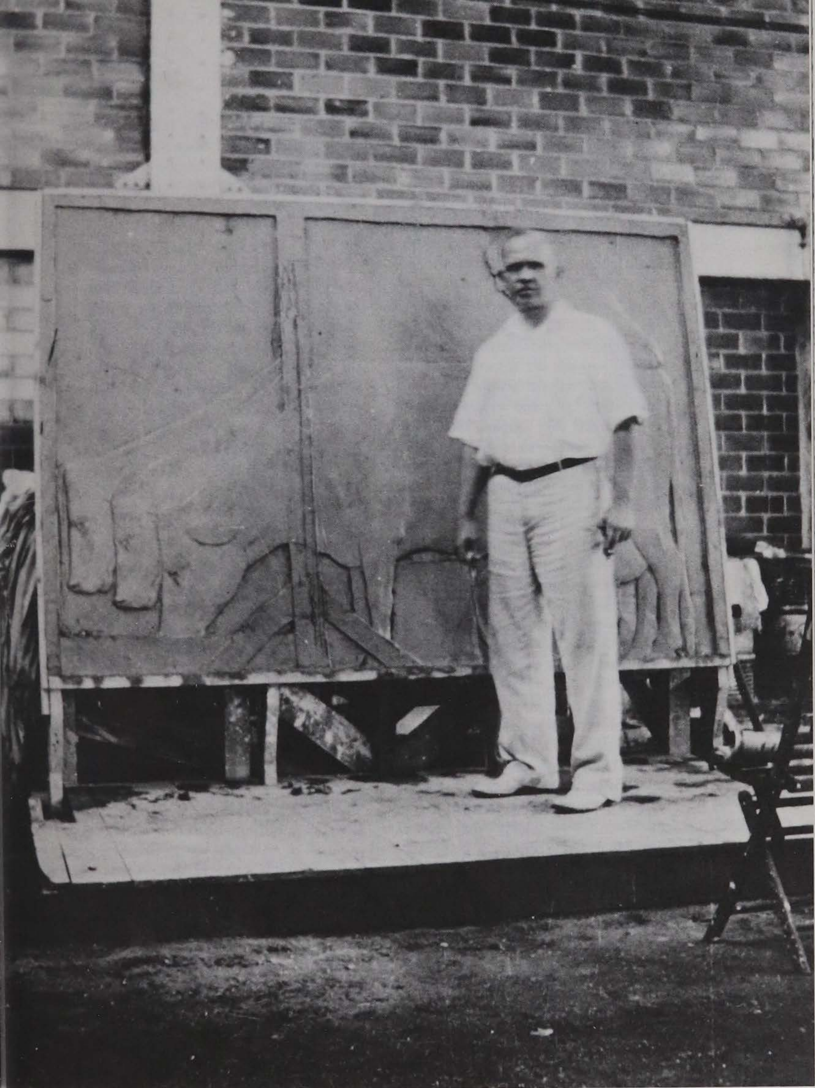
PETERSEN IN THE UNIVERSITY OF IOWA ARMORY, 1934. CPP
