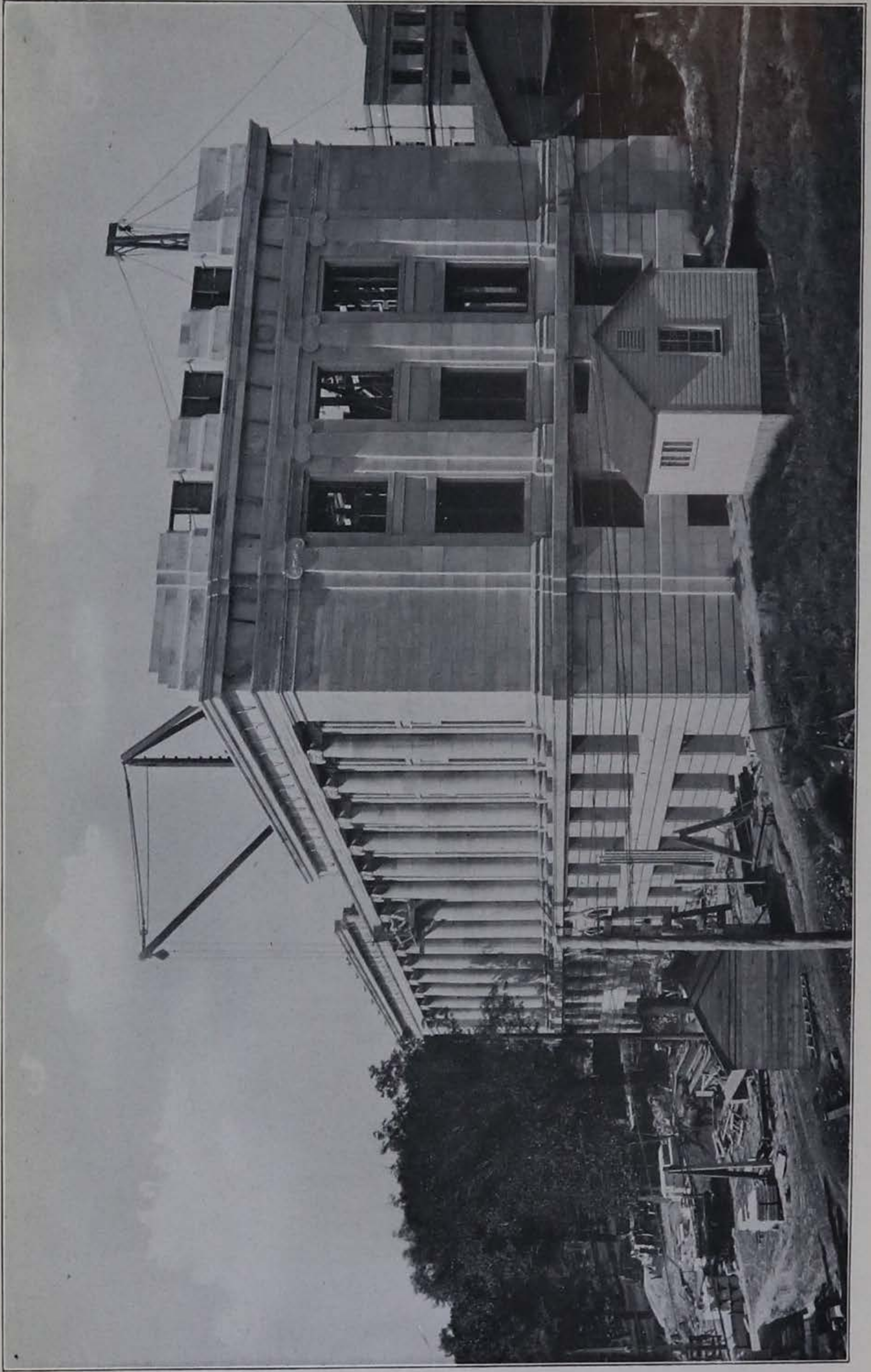
THE NEW PHYSICS BUILDING, NOW UNDER CONSTRUCTION
