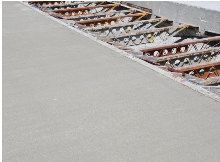
Figure 65. Bridge Deck Concrete Placement, Cured Concrete Bridge Deck, and Inclined Bar Receiver Holes
