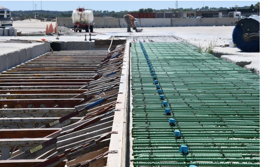
Figure 64. Installation of Bridge Deck Reinforcement, Rebar Cage, Formwork, and Receiver
