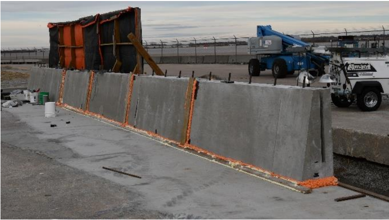
Figure 70. Precast Concrete Barrier Placement Process
