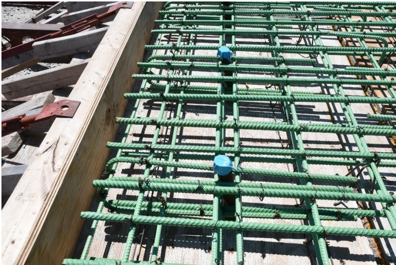
Figure 64. Installation of Bridge Deck Reinforcement, Rebar Cage, Formwork, and Receiver
