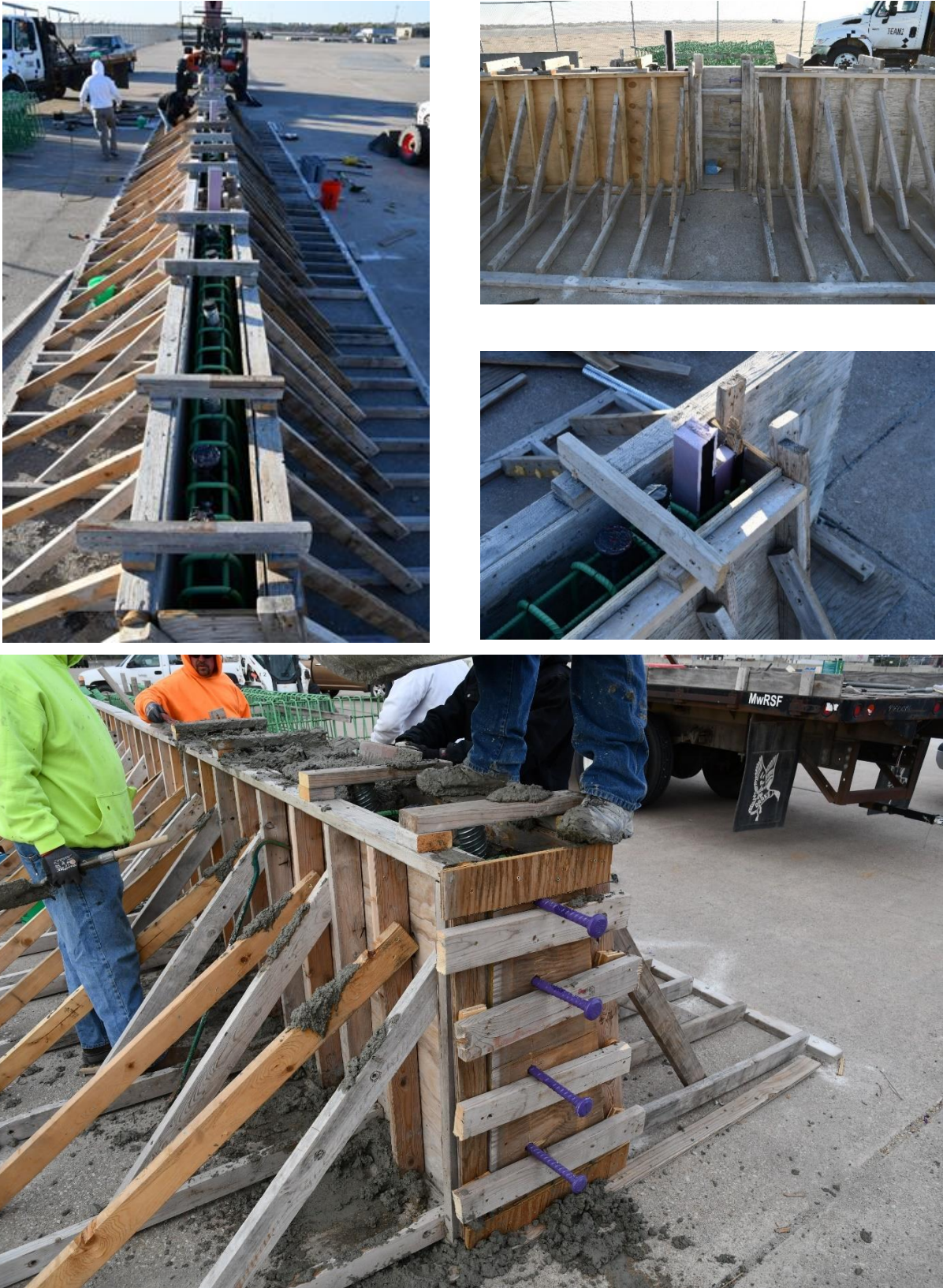
Figure 62. Precast Concrete Barrier Construction Prior to and During Concrete Casting
