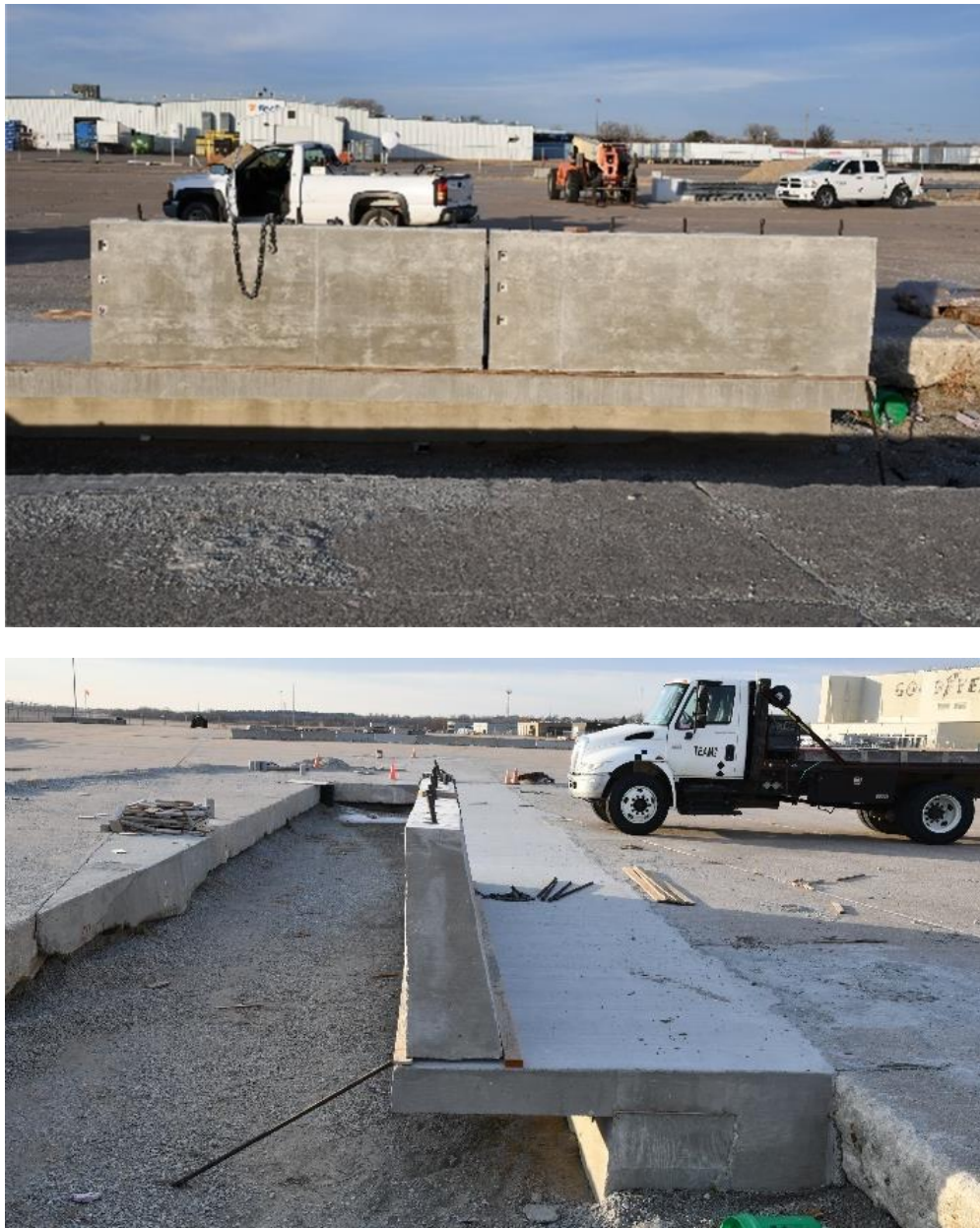
Figure 68. Precast Concrete Barriers on Bridge Deck
