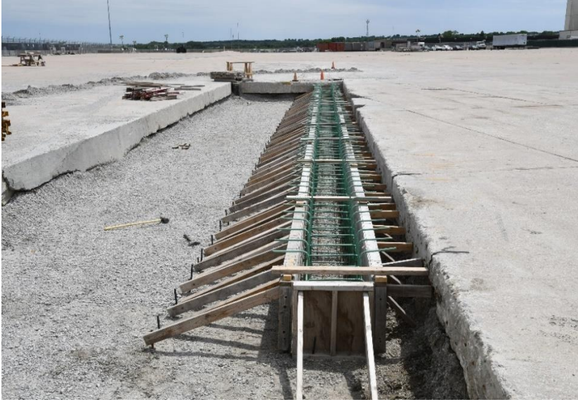
Figure 63. Grade Beam and Anchor Beam Installation
