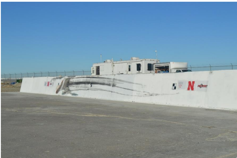
Figure 89. Overall System Damage, Test No. ABCBRM-1
