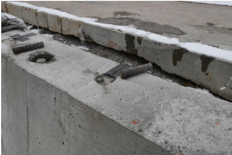
Figure 71. Inclined Bars After Grout Application
