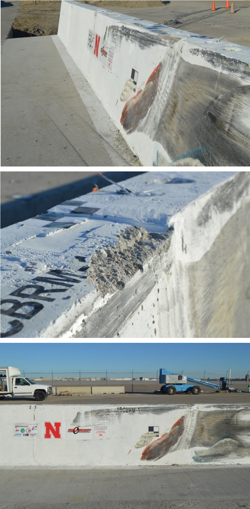
Figure 90. System Damage, Downstream Gouge Details, Test No. ABCBRM-1
