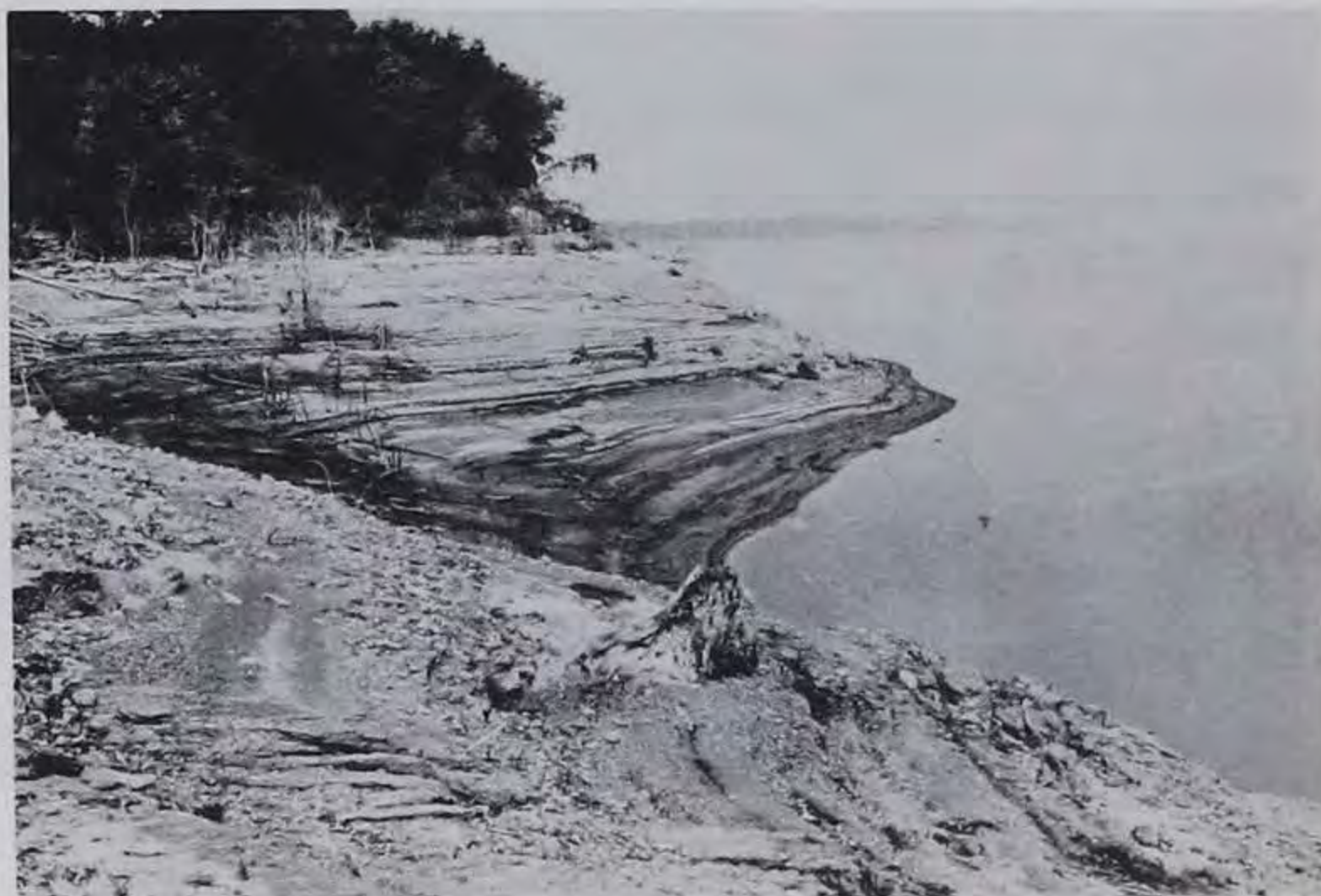
Fig. 7. Erosion slopes near Red Rock Lake dam with water at conservation pool level; high water reached approximately 50 feet higher as shown by erosion line on slopes; photographed 15 August 1974.
