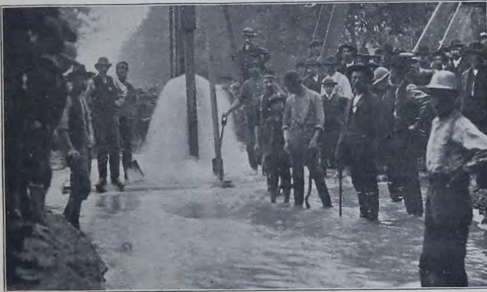
FIG. 43. Artesian well in glacial drift, Belle Plaine, Iowa. Jumbo while uncontrolled.
