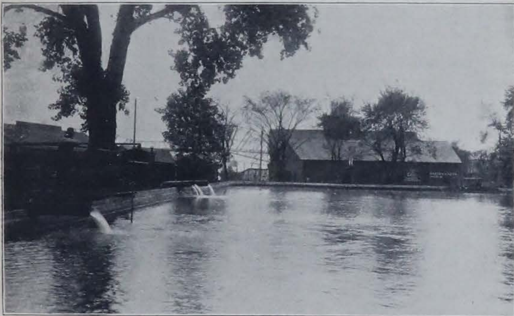
FIG. 40. Reservoir at Clinton, Iowa, fed by artesian wells. The smallest stream, the second on the left, is of filtered water from the Mississippi river.
