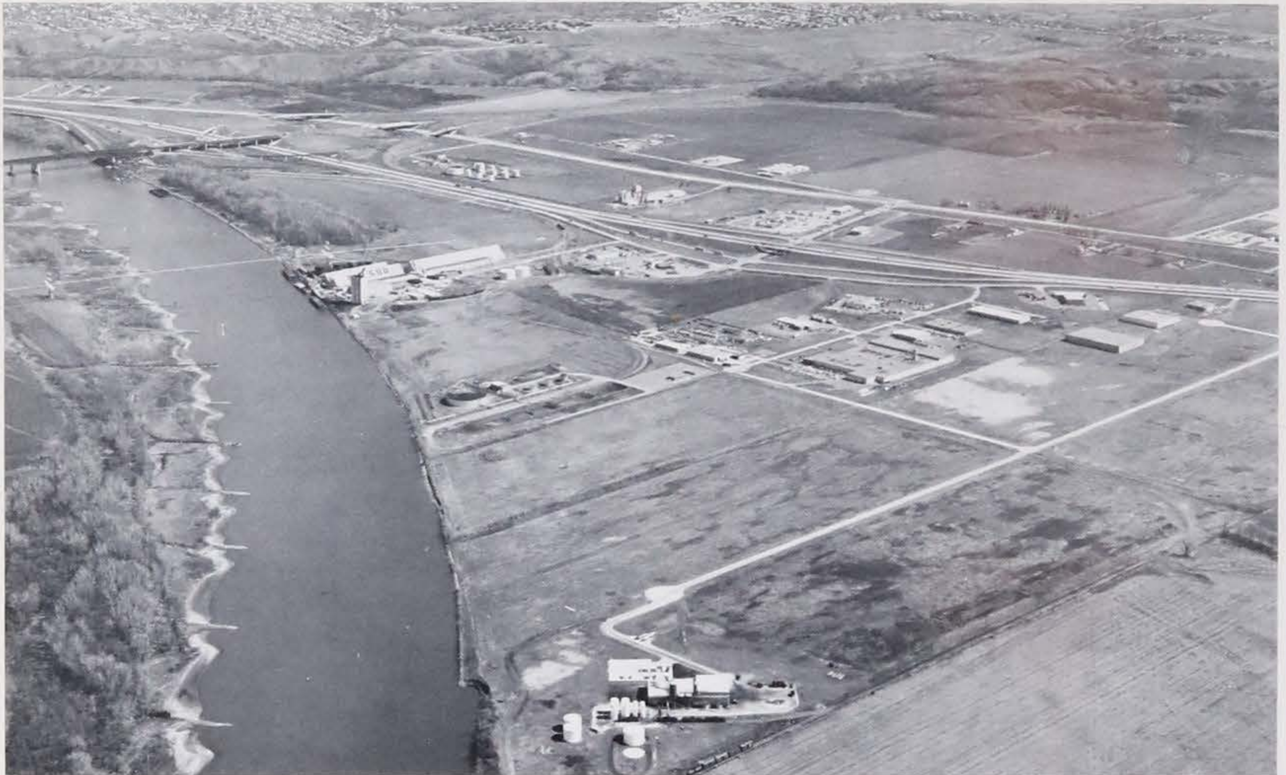
Industrial Interchange, Missouri River at Sioux City.
