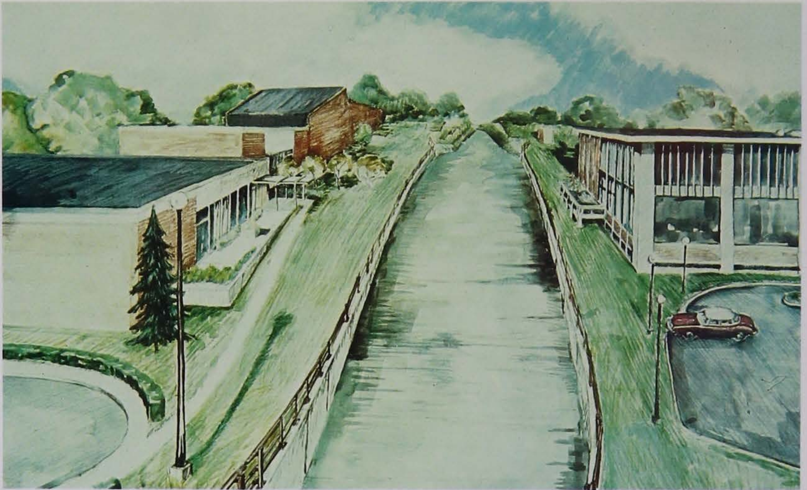
Artist's drawing of a portion of the Marshalltown project, showing architectural blending of floodwalls with surrounding environment.
