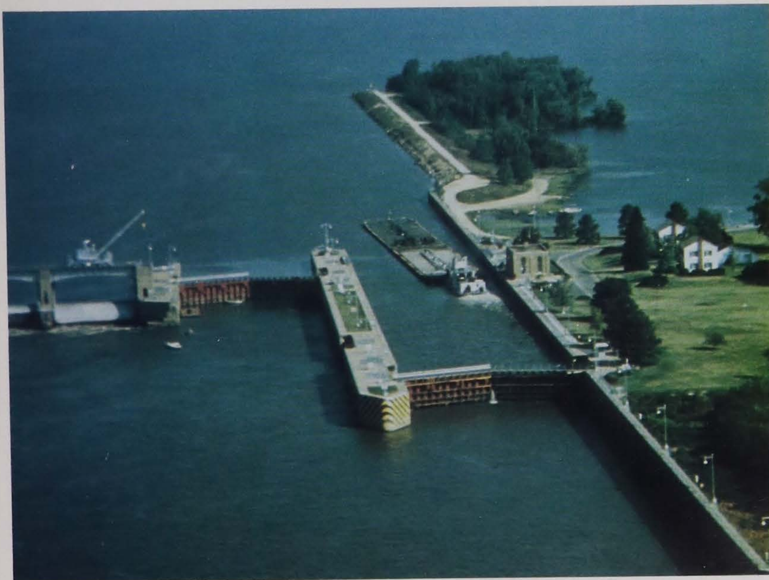
Mississippi River Lock and Dam No. 13, upstream from Clinton.
