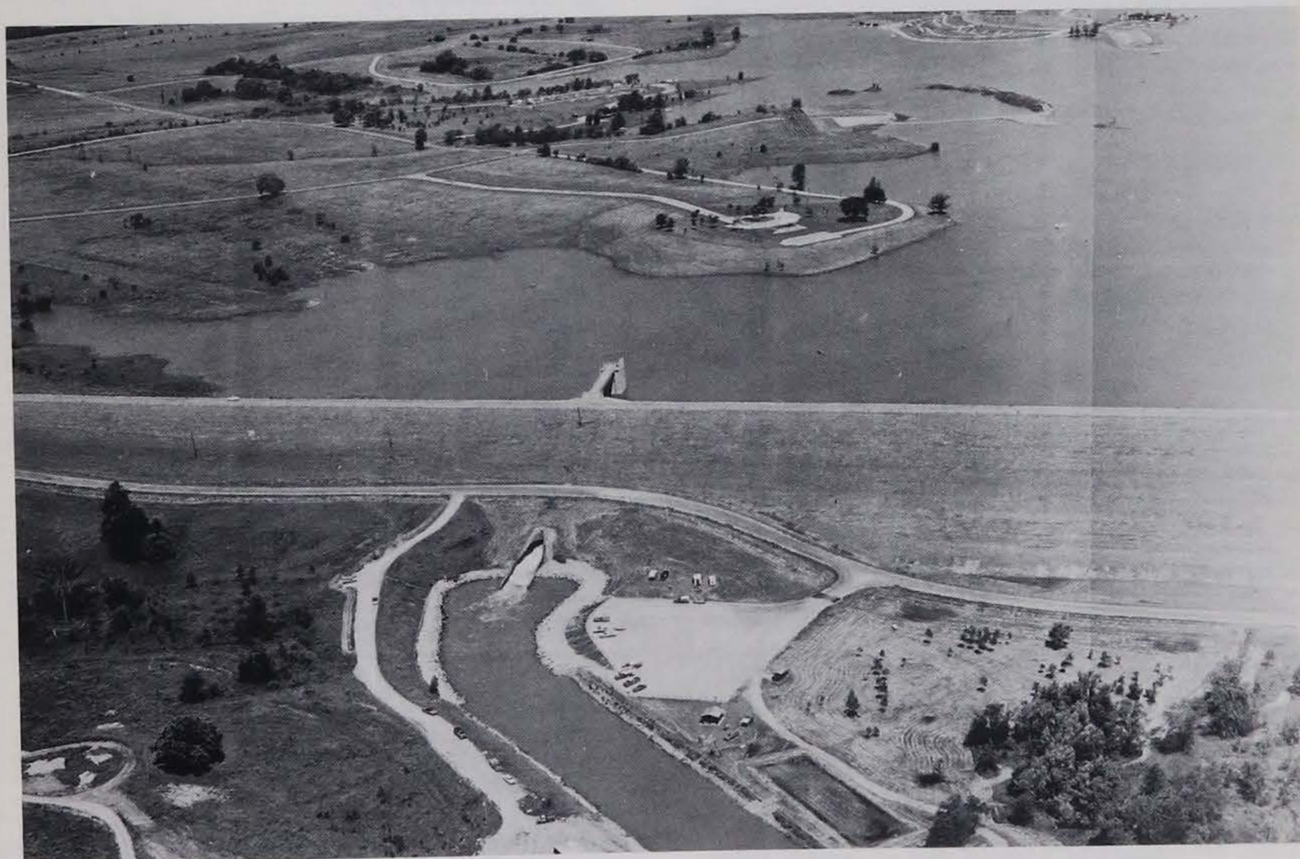
Downstream face of Rathbun Dam.
