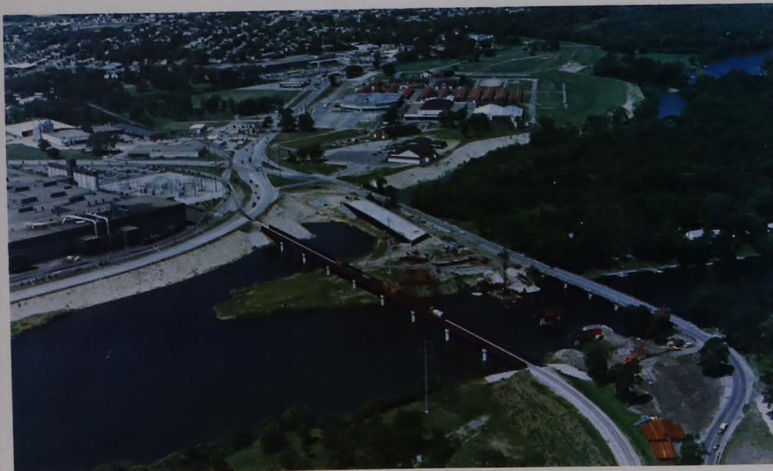
Levees and new railroad bridge, Waterloo project.
