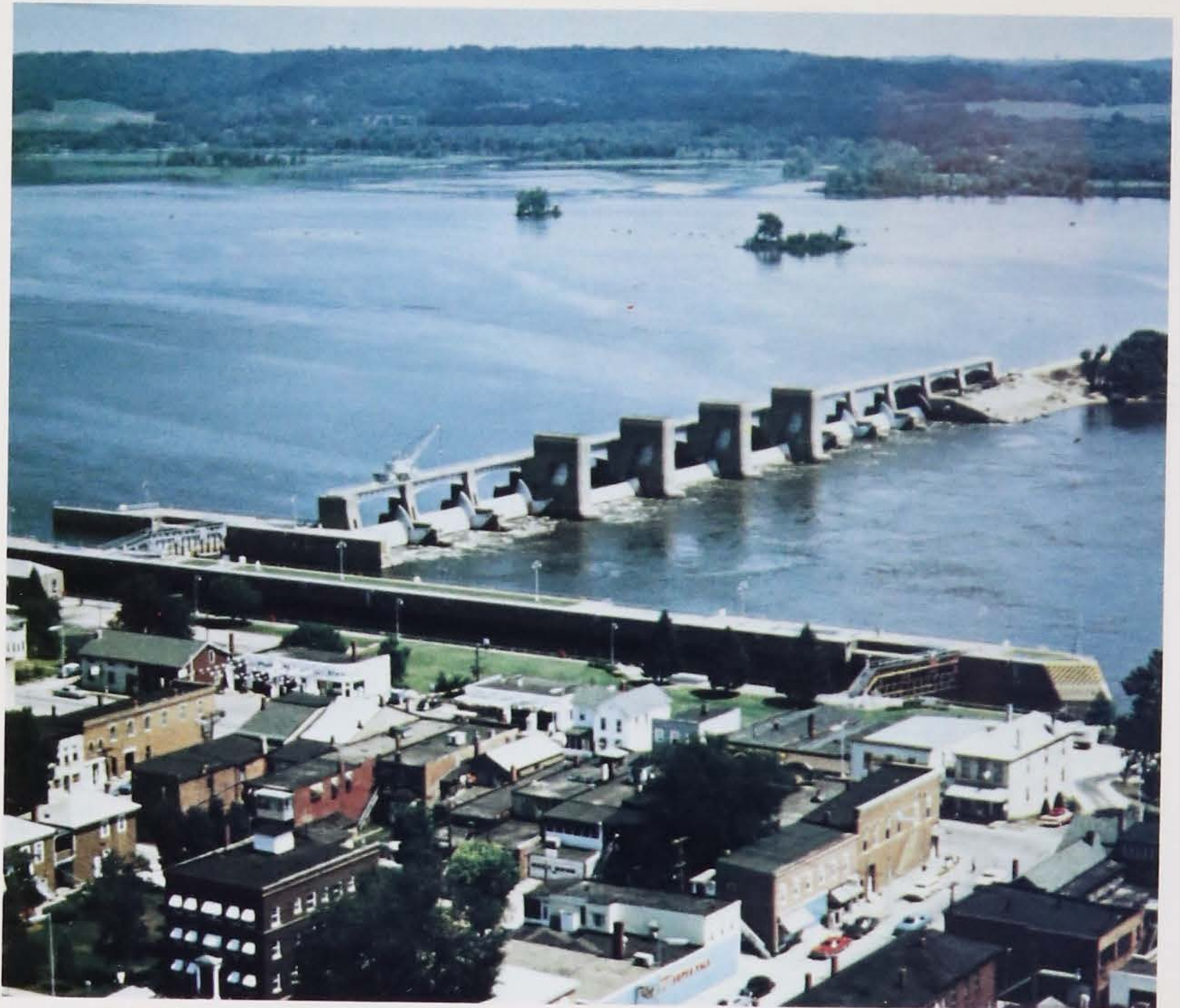
Mississippi River Lock and Dam 12 at Bellevue.
