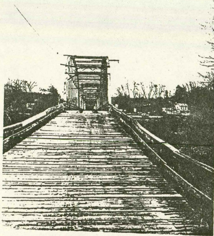
Fig. 5. West approach of existing bridge. View to the east.
